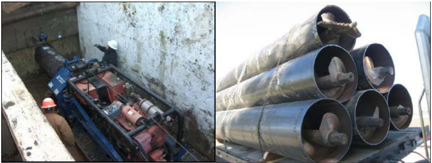
Figure 4-31: Auger Bore and Jack
