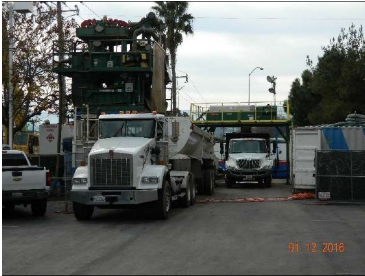
Figure 4-39: MT equipment to process cuttings and provide slurry
