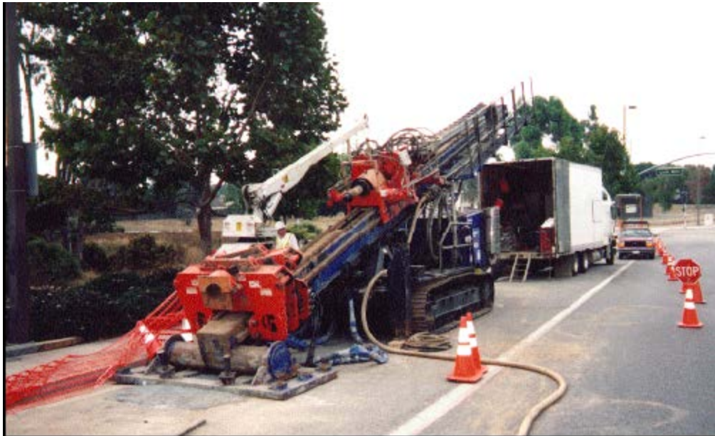
Figure 4-36: HDD Rig
