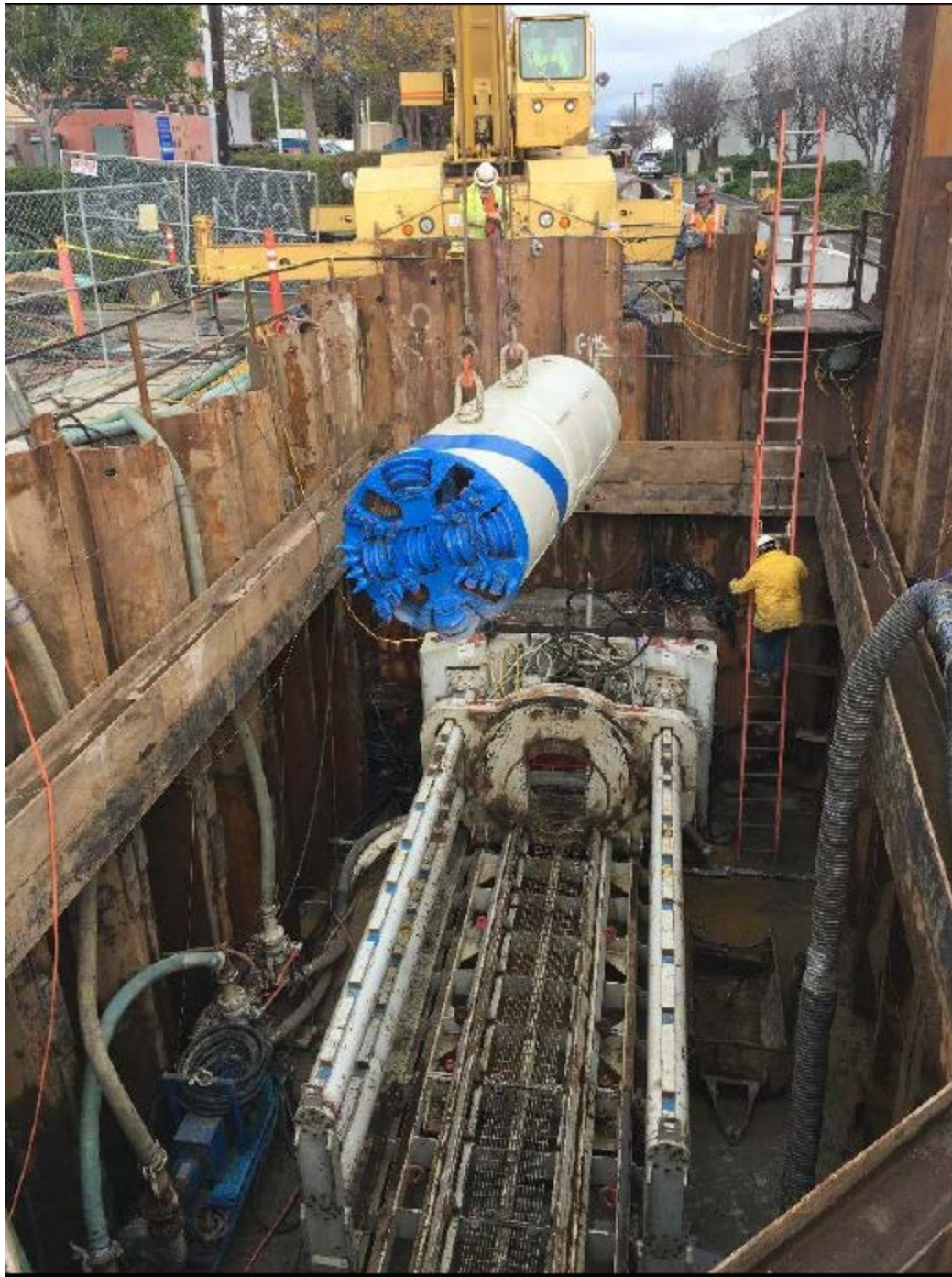
Figure 4-38: Microtunnel jacking pit preparation and MTBM positioning
