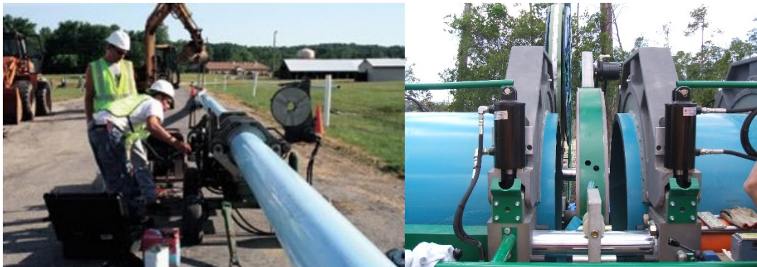
Figure 4-3: Butt Fusion Machine for FPVC
