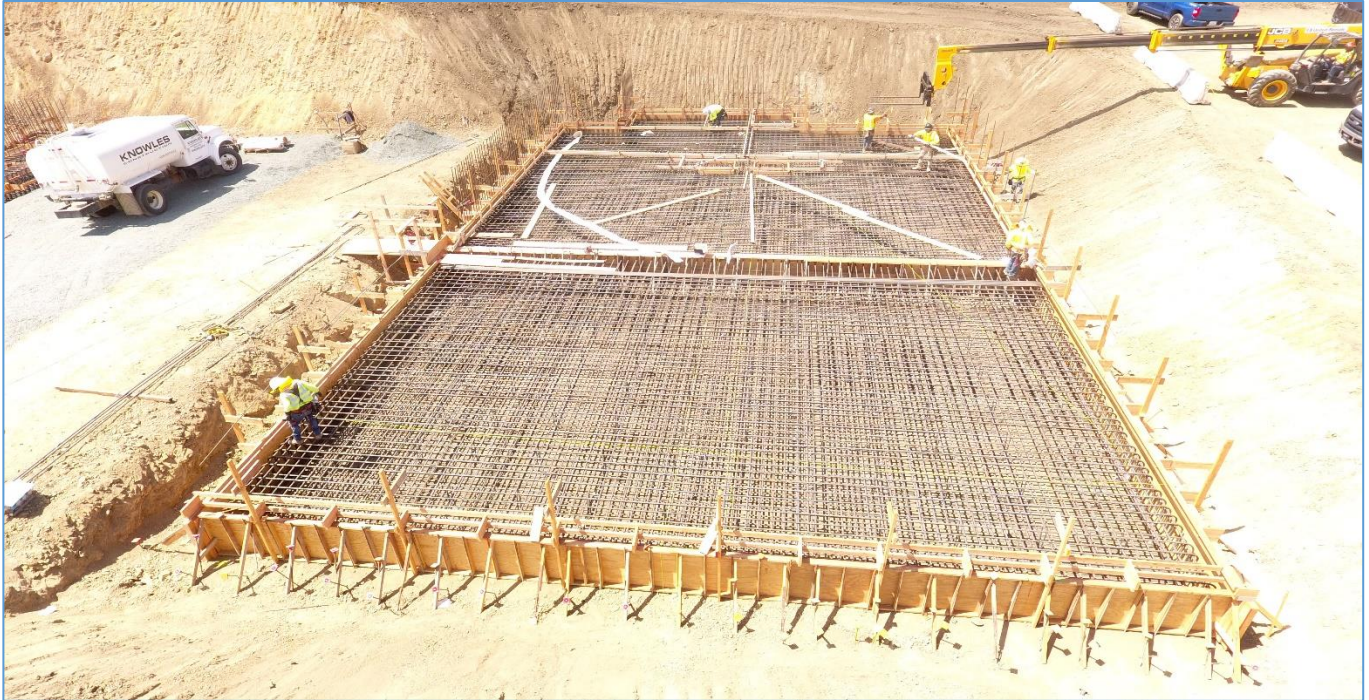
August 5, 2020 – Looking north at BNR basins slab-on-grade forming and rebar.
