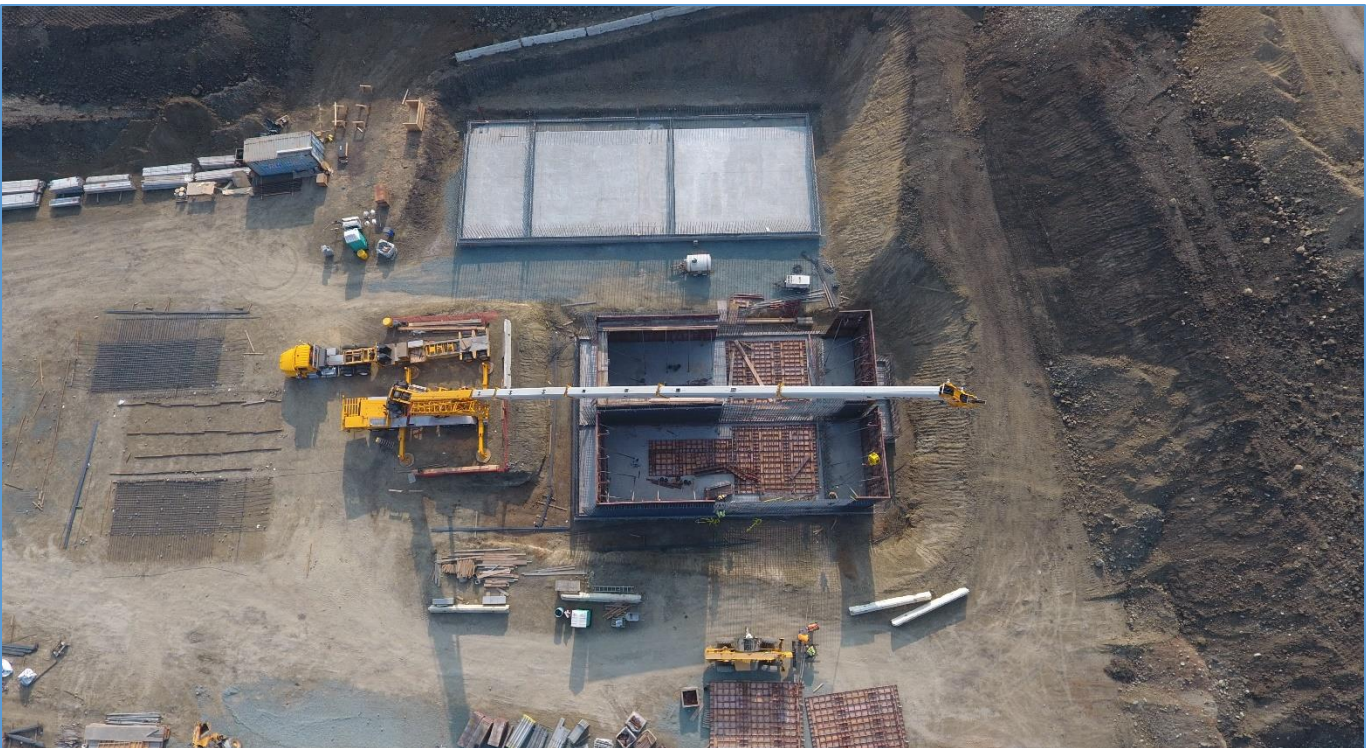
Sept. 15, 2020 – Looking down at BNR basin – 110 ton crane flying in wall rebar curtains (pre-tied on ground)
