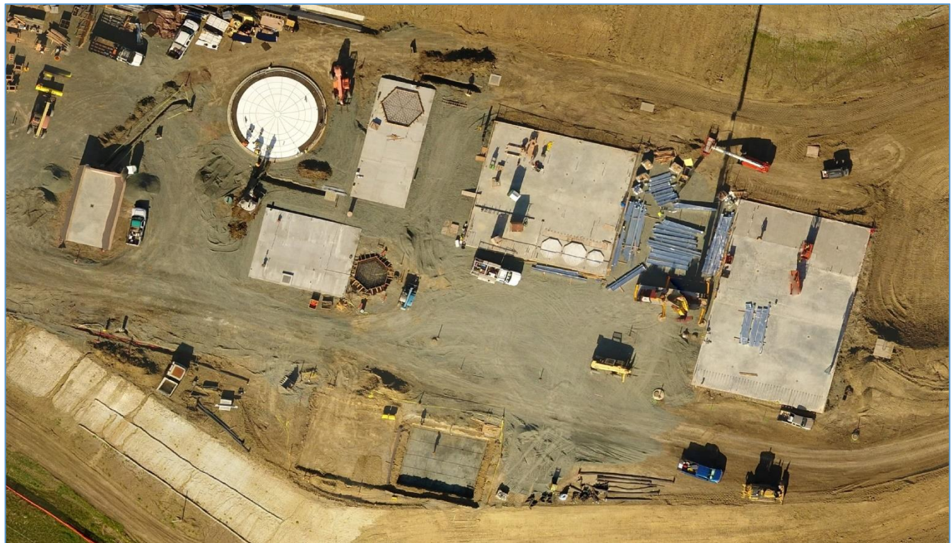
March 31, 2021 – (L to R): Wash Rack slab and CMU walls, Product Water Tank erection, IPR/Outfall Pump Station slab, Balancing Tank slab forms and rebar, Calcite Contactor slab, RO/UV Bldg slab, and Maint Bldg slab with steel erection. Also note Chemical Facility containment areas over-excavation and subgrade preparation (lower frame of photo).
