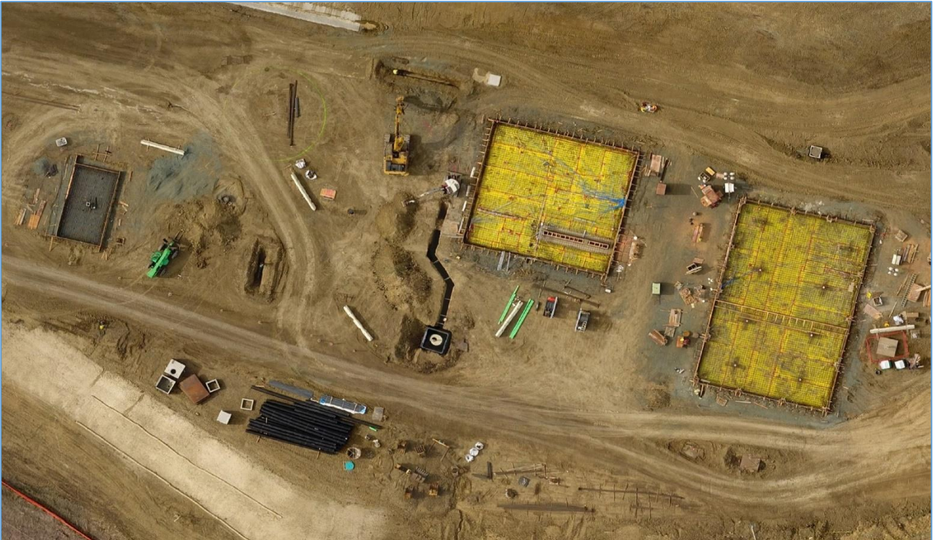
January 6, 2021 – (L to R): Wash Rack slab forms and rebar, Product Water Tank layout, IPR/Outfall Pump Station and Balancing Tank slabs not started, Calcite Contactor slab not started, RO/UV and Maint Bldg slab forms and rebar, etc.
