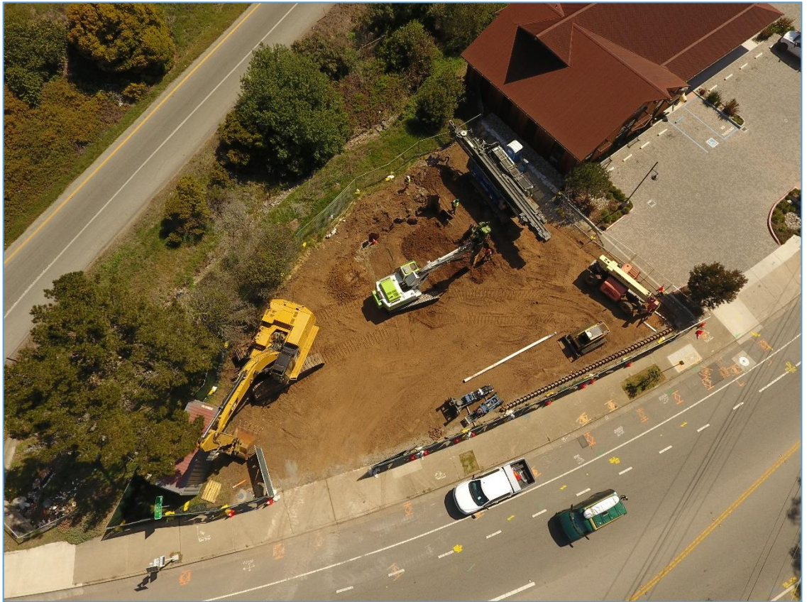
March 31, 2021 – Looking down – Pump Station B site, installing shoring & dewatering systems.
