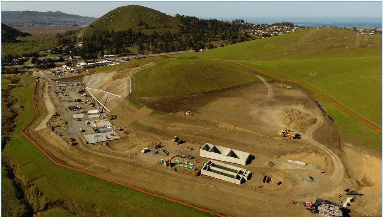
March 31, 2021 – Looking S.W. – BNR and SHT Basins (both structures completed, leak tested, backfilled)
