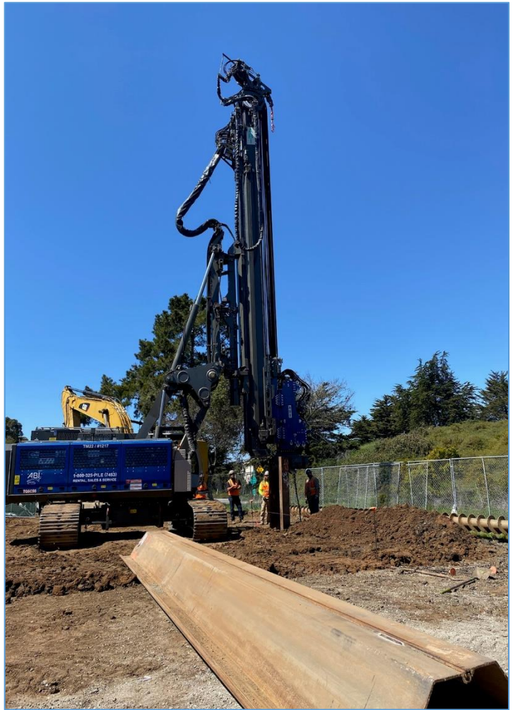
Pump Station B (sheet pile shoring installation)
