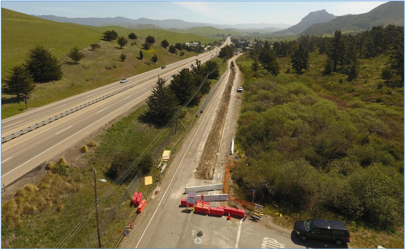
March 31, 2021 – Looking S.E. – Quintana at La Loma – Road Closed detour, pavement removal, HDPE pipe segments fused/welded and stored along road for upcoming installations (left side of road).
