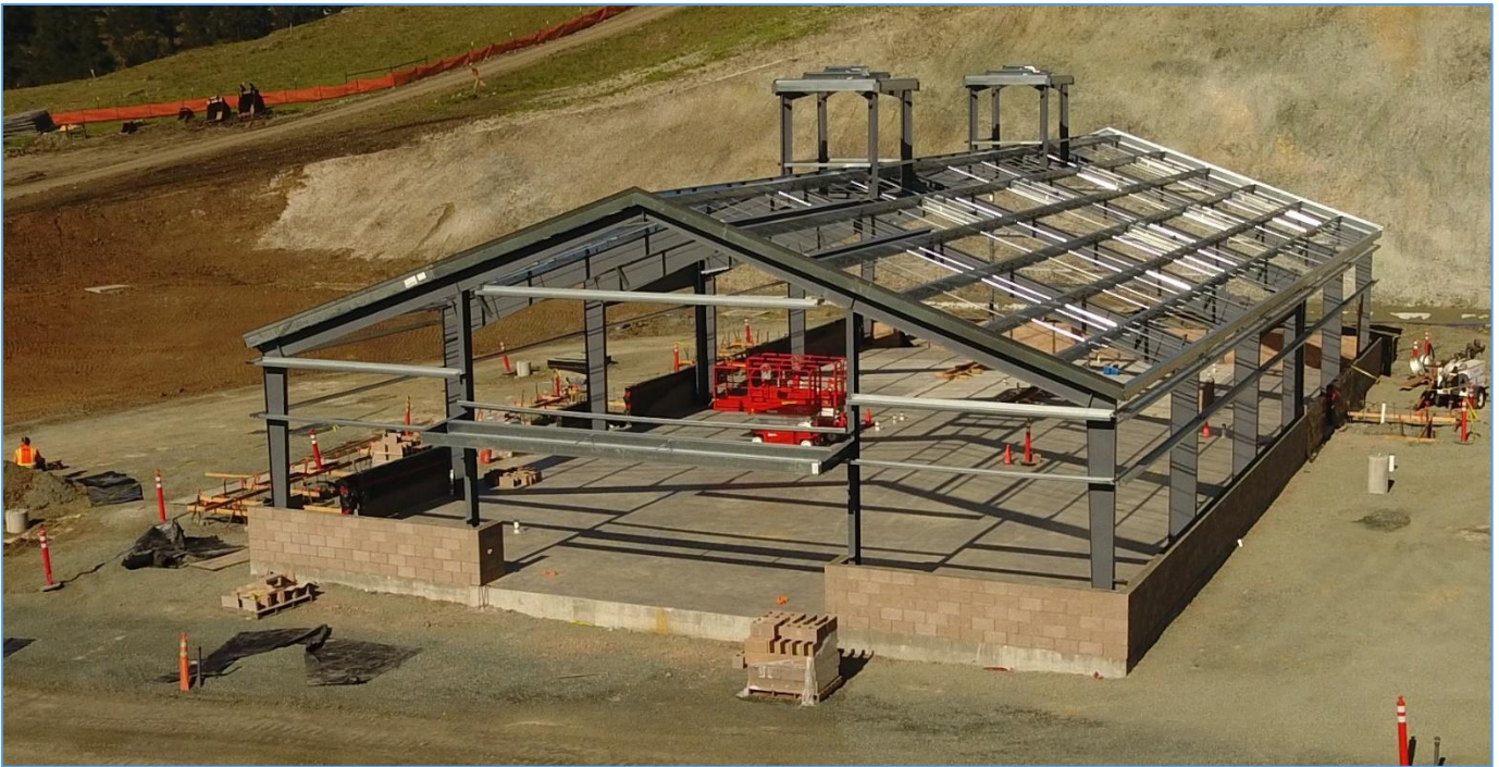
March 31, 2021 – Operations Building (steel erection and CMU wainscot wall)
