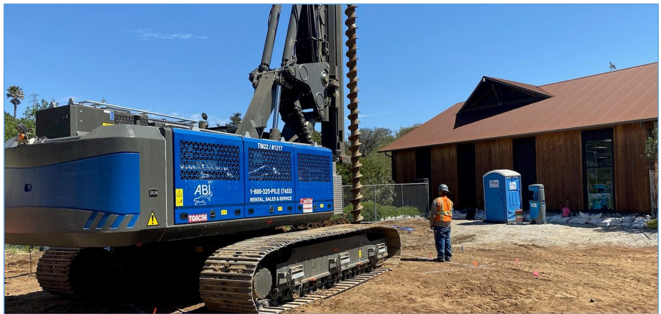
Pump Station B (drilling pilot holes for sheet pile shoring system)
