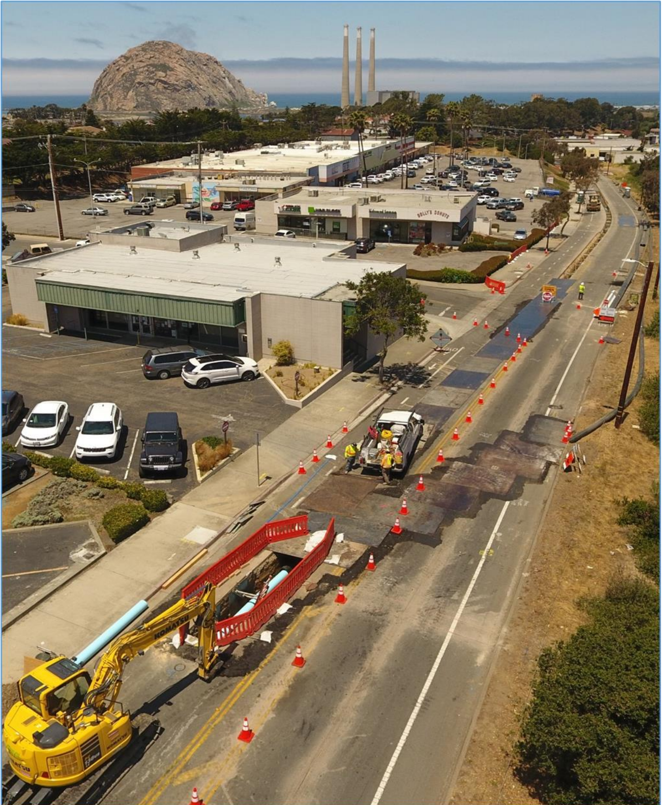
June 30, 2021 – Segment 5 (Quintana - Main to Morro Bay) – 12-inch Water Relocation/Tie-in, and temp bypass pipe
