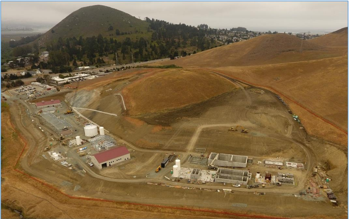
June 30, 2021 – Looking S.W. – North Site (note: MBR slab and cassette tanks, Headworks facility, Elect. Facility slabs)
