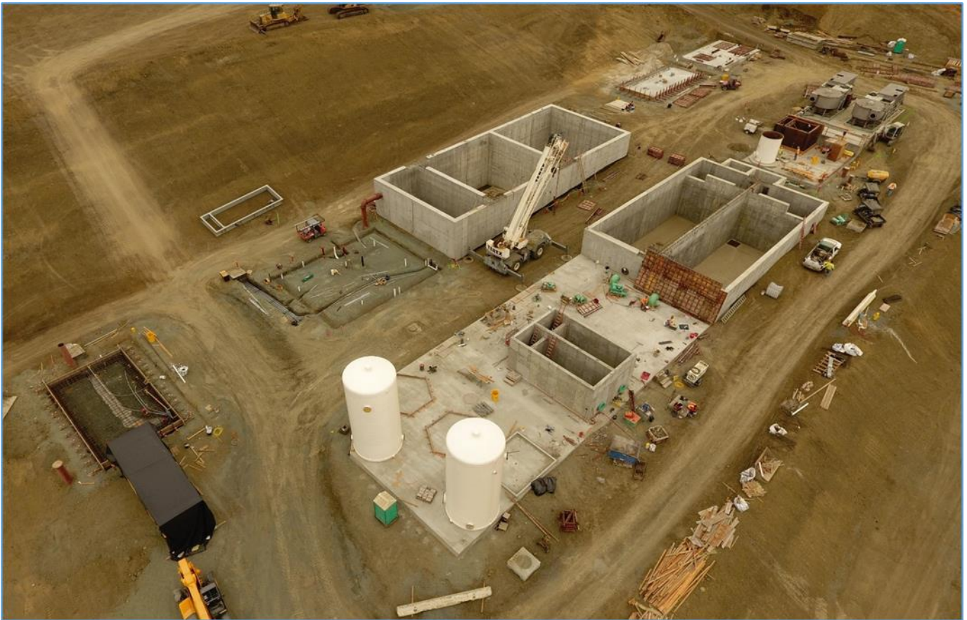
June 30, 2021 – North Site (L to R): SAFE (rebar), Dewatering (subgrade), MBR, SHT, BNR, Elect. Bldg., Headworks.
