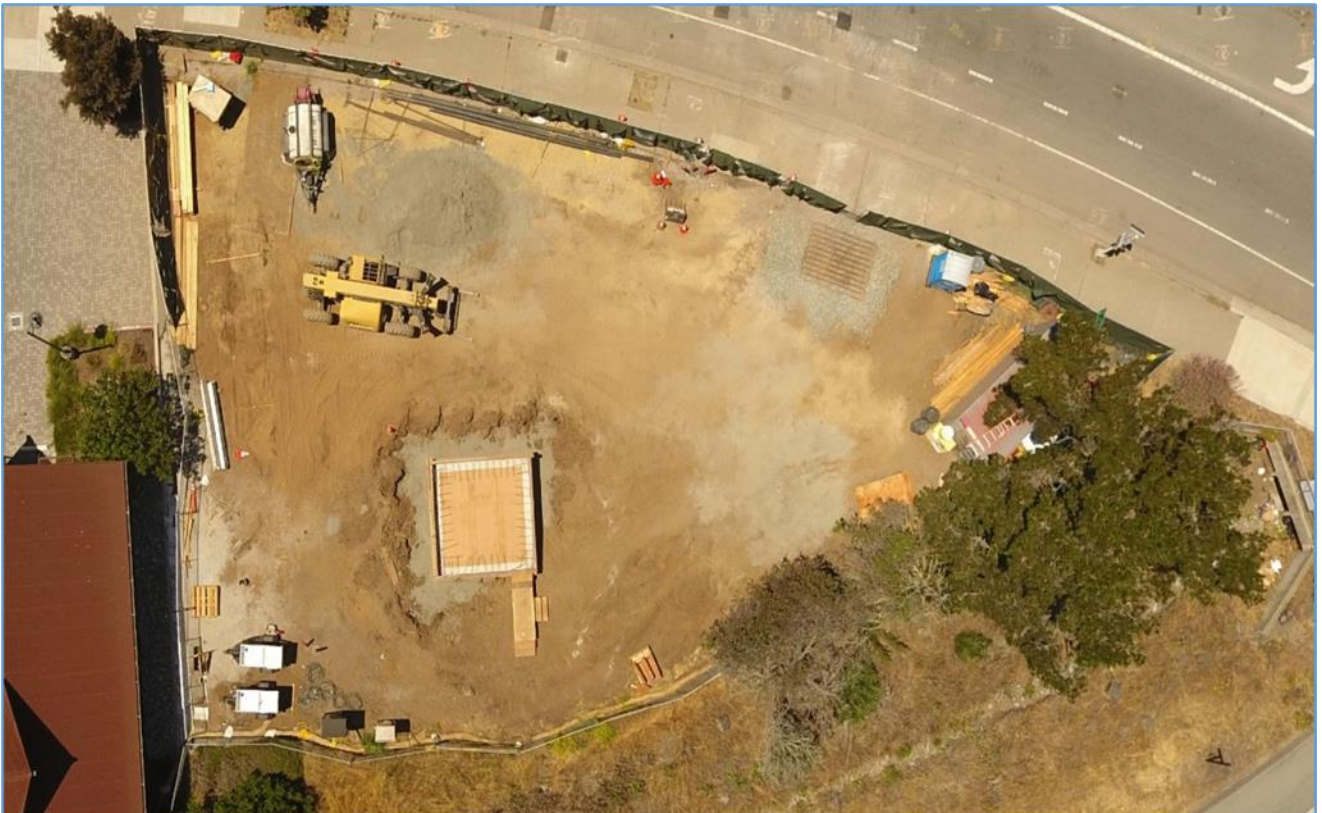
June 30, 2021 – Pump Station B (note deep wet well structure completed and sheet pile shoring system removed)
