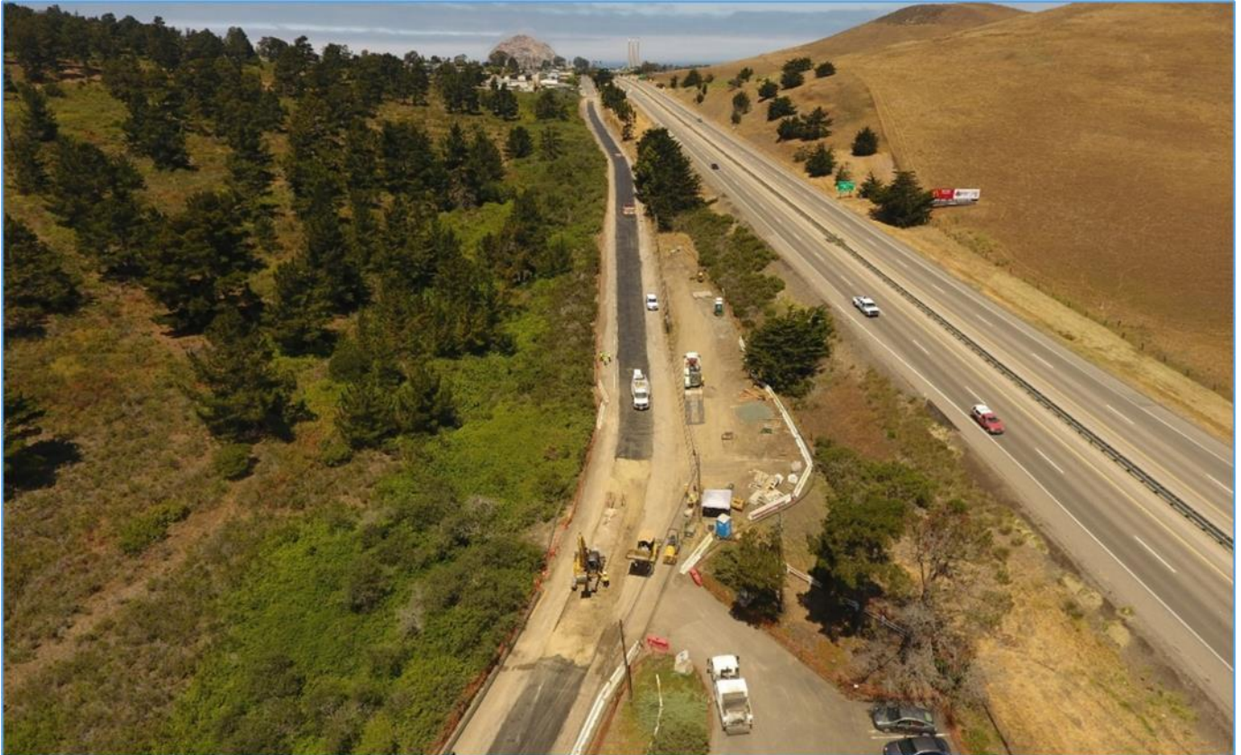
June 30, 2021 – Segment 7 (Quintana – La Loma to South Bay) – Joint Trench, IPR, Waterline Relocation work on-going
