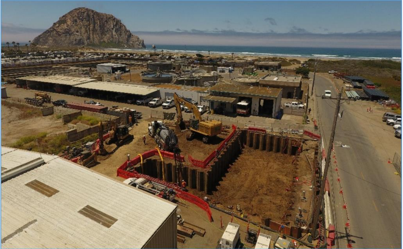
June 30, 2021 – Pump Station A (note sheet pile shoring system and deep wet well excavation in progress)
