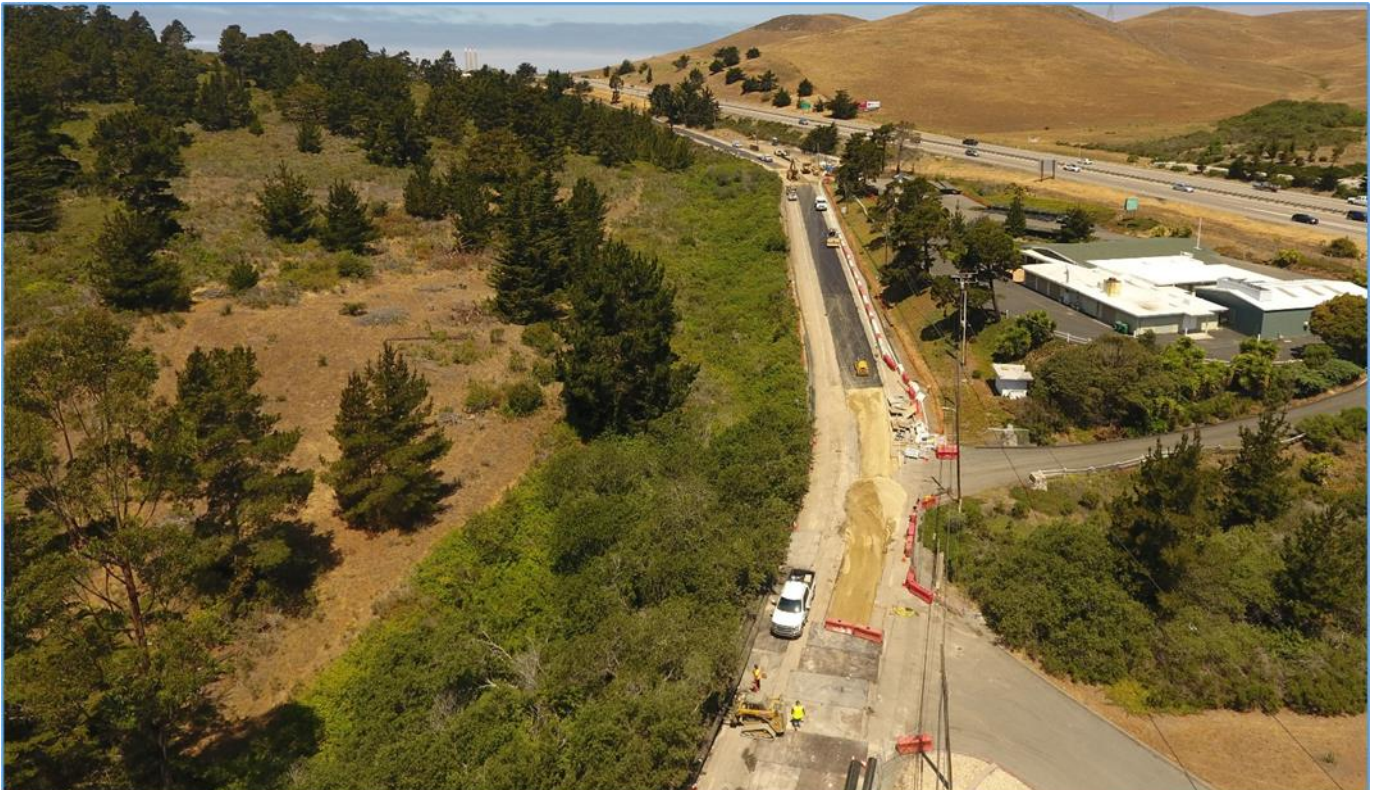
June 30, 2021 – Segment 7 (Quintana – La Loma to South Bay) – Joint Trench, IPR, Waterline Relocation work on-going
