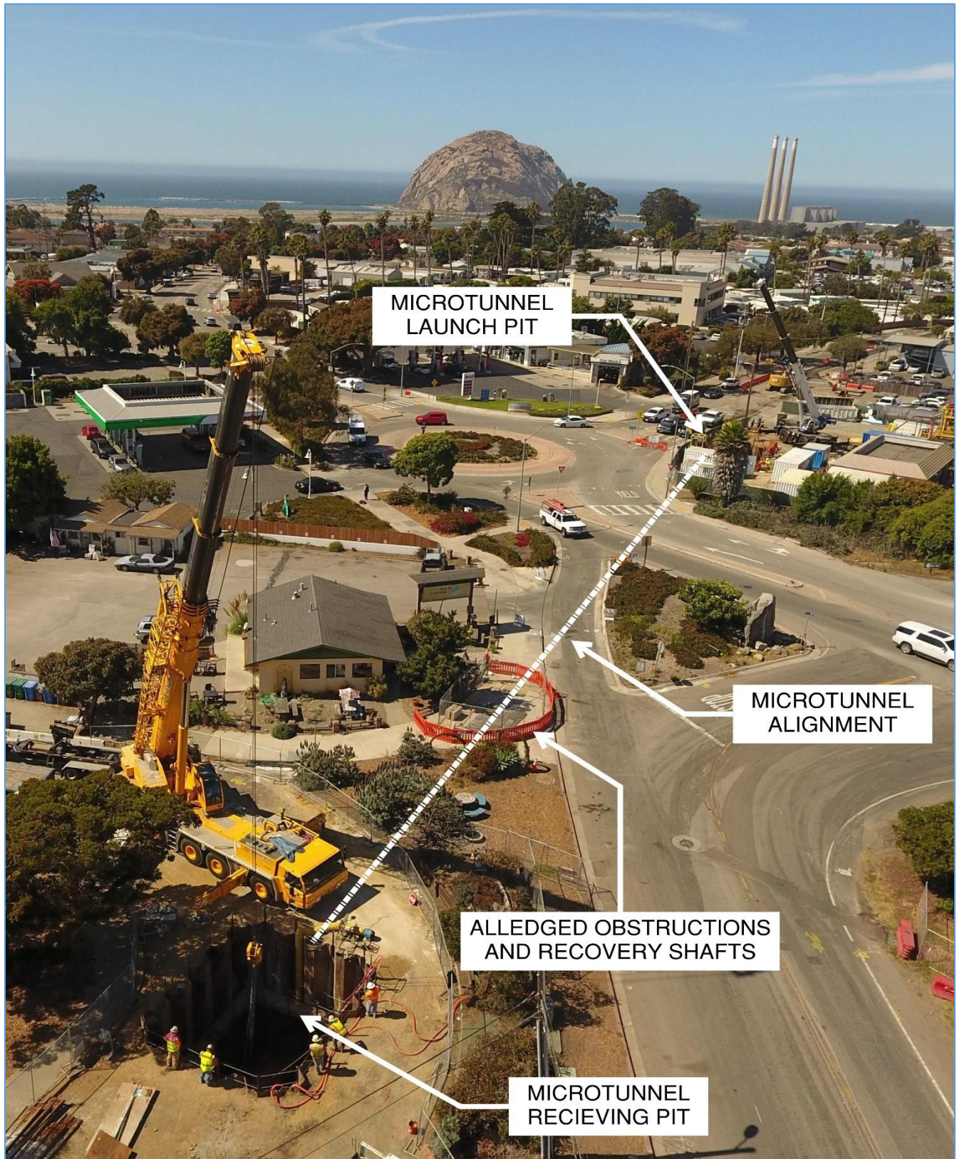
Sept. 28, 2021 – Morro Bay Blvd Roundabout Microtunnel (removing MTBM from Receiving Pit with Bragg Crane)
