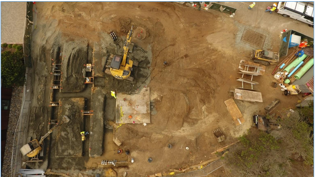
Sept. 27, 2021 – Pump Station B (Electrical Building underslab conduit and stub-up installations on going)
