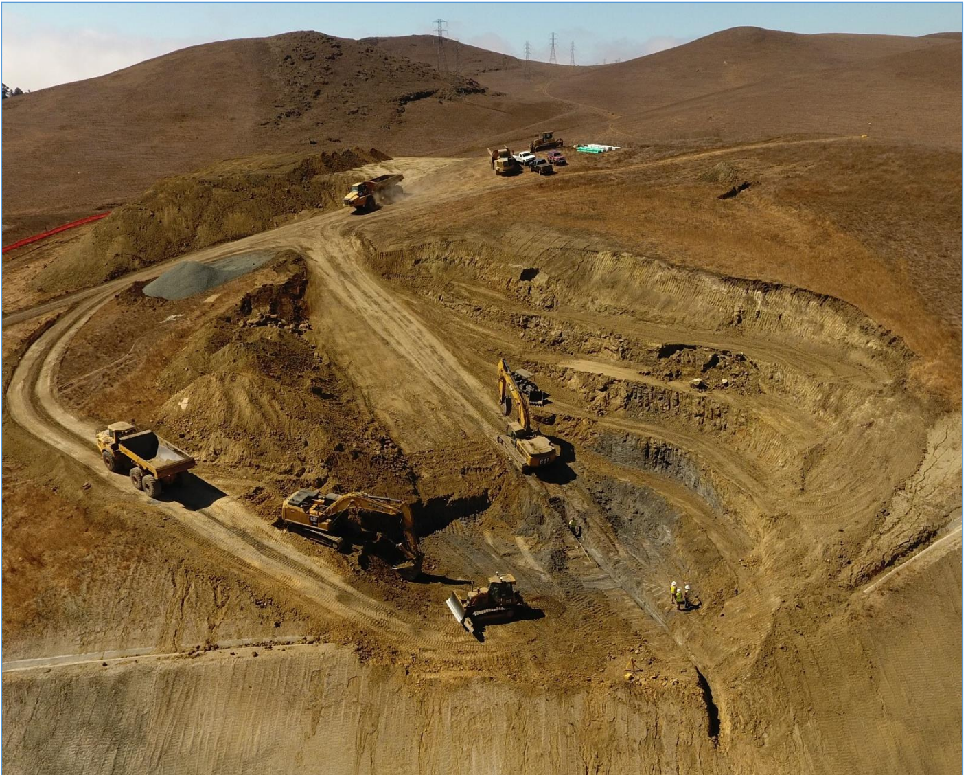
Sept. 22, 2021 – Landslide Remediation: removing loose material, benching into competent subgrade, installing subdrain.
