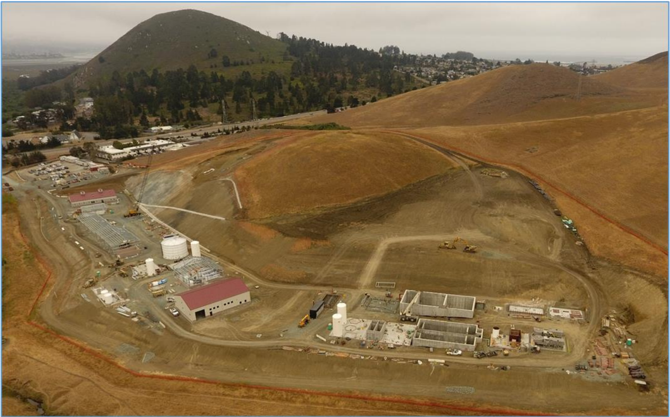
July 1, 2021 – Looking S.W. – North Site (note: MBR slab/tanks, Headworks, Elect. Bldg, BNR and SHT Basins).
