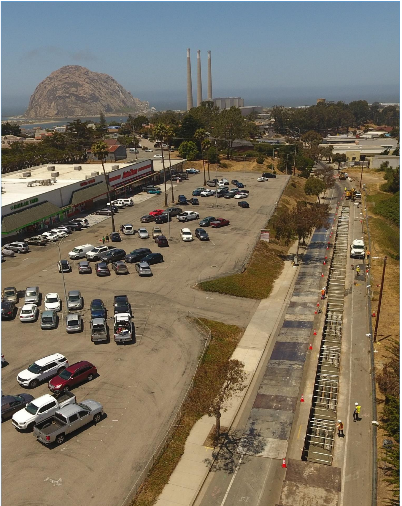
July 21, 2021 – Segment 5 (Quintana - Main to Morro Bay) – Joint Trench piping, shoring, and CLSM placement
