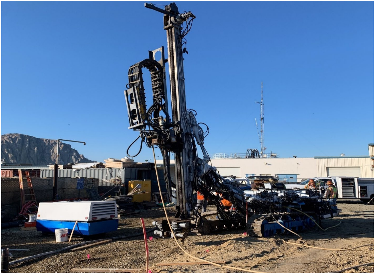
Soil improvements at Pump Station A Site
