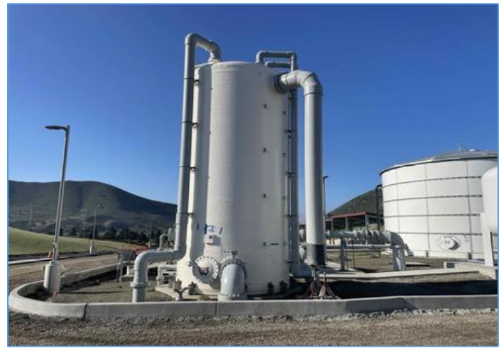
March 31, 2022 – Outfall Balancing Tank
