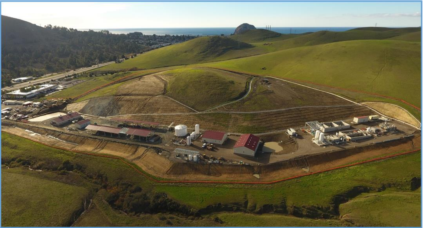
January 1, 2022 – Looking West – Entire Site (Ops Bldg, Maint Bldg, RO/UV Bldg, MBR Plant, Headworks, Etc.)
