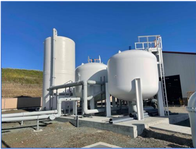
March 31, 2022 – Calcite Treatment Facility
