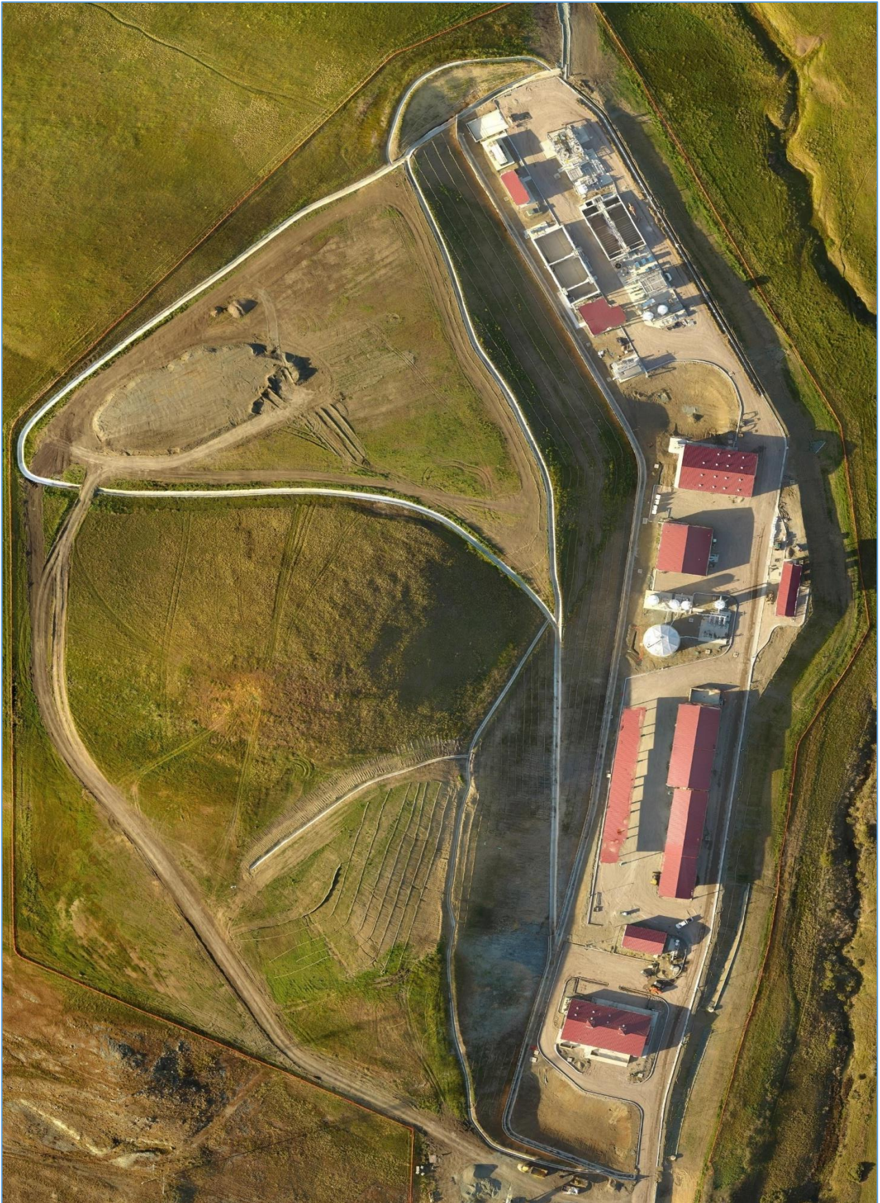
March 31, 2022 – Looking down at entire WRF Site.
