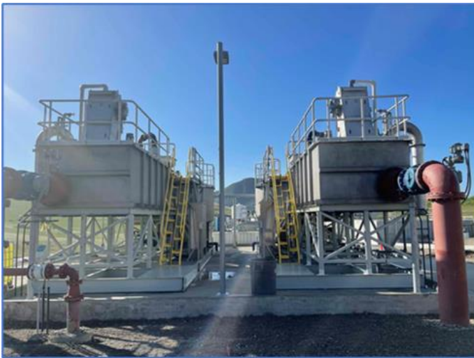
March 31, 2022 – Headworks Skids
