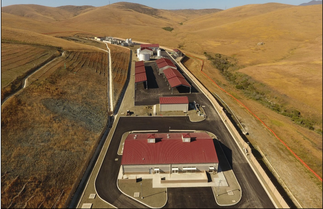
June 6, 2022 – Looking North – South Site (Operations Building, Storage, Parking Canopies)
