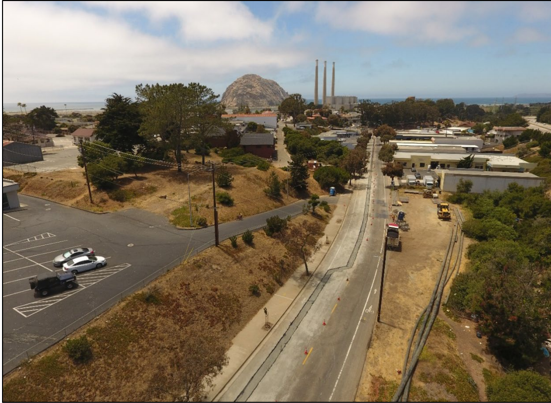
March 31, 2022 – Segment 5 (IPR Pipeline Installation along Quintana Rd)
