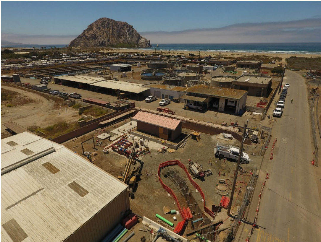
June 30, 2022 – Pump Station A (Aboveground Piping Progress / Electrical Bldg Structure Complete)
