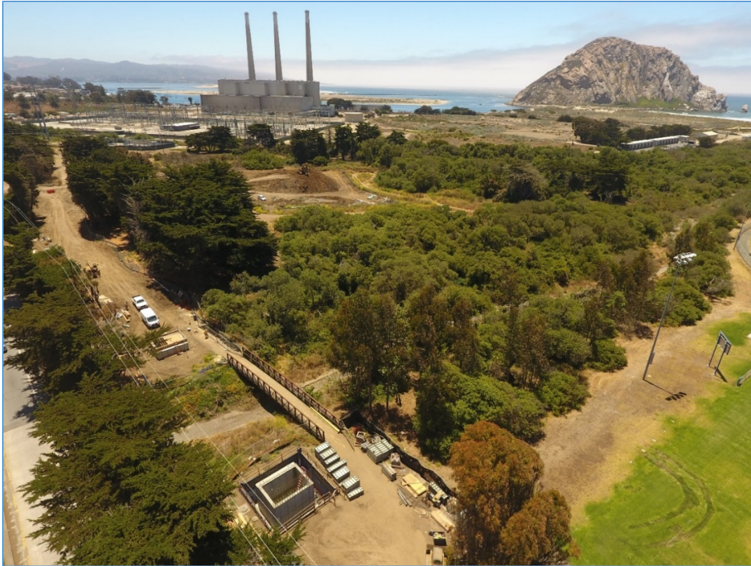
June 30, 2022 – Segment 3 (Utility Bridge North and South Abutment Construction Progress)
