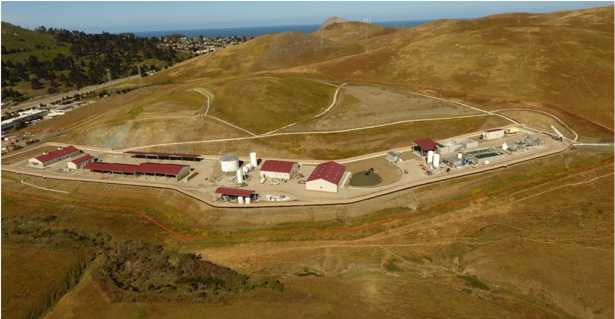
May 9, 2022 – Entire Site Pre-Pavement (Ops Bldg, Maint Bldg, RO/UV Bldg, MBR Plant, Headworks, Etc.)
