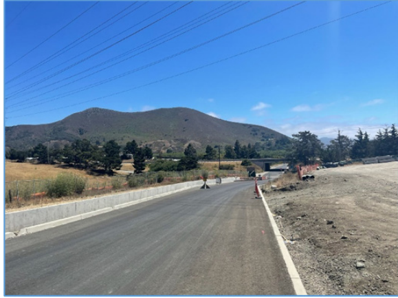
June 30, 2022 – WRF Site Driveway
