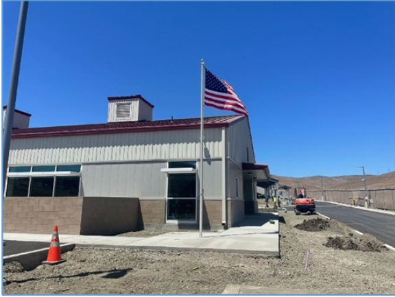
June 30, 2022 – Operations Building Exterior
