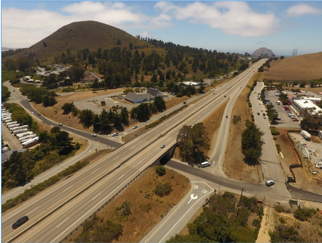
June 30, 2022 – Segment 8 – Point of connection between projects (Anvil > FBV)
