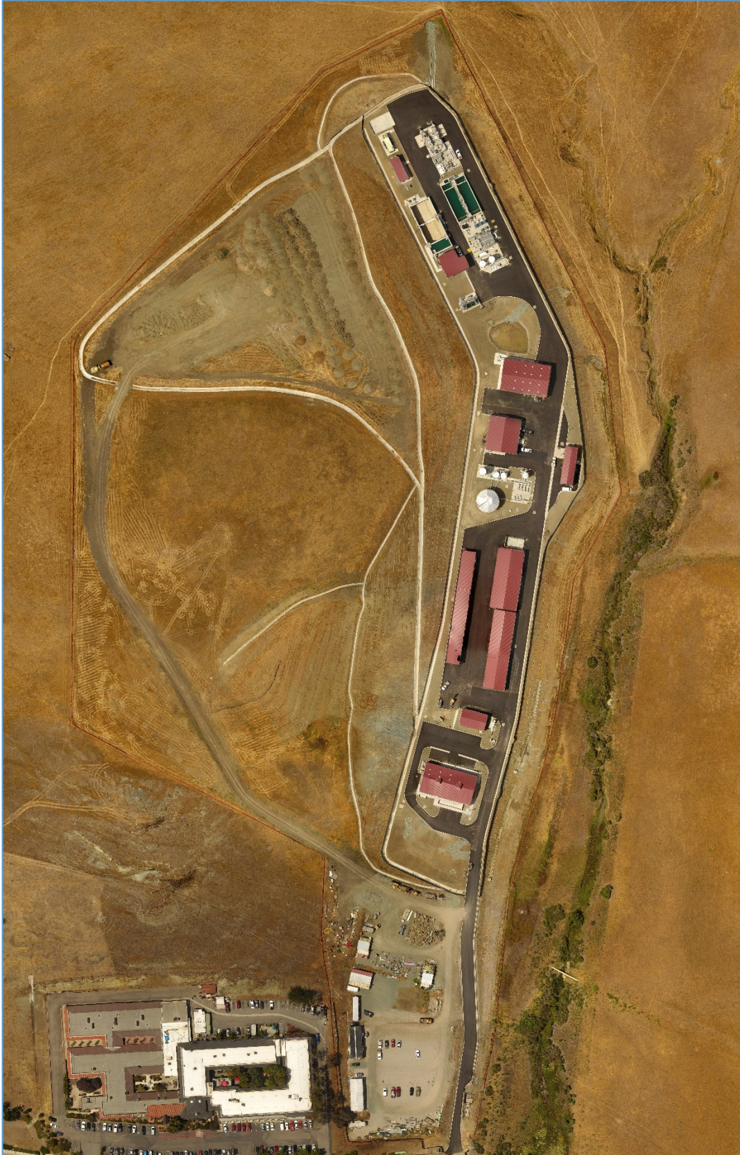
March 31, 2022 – Looking Down at Entire WRF Site
