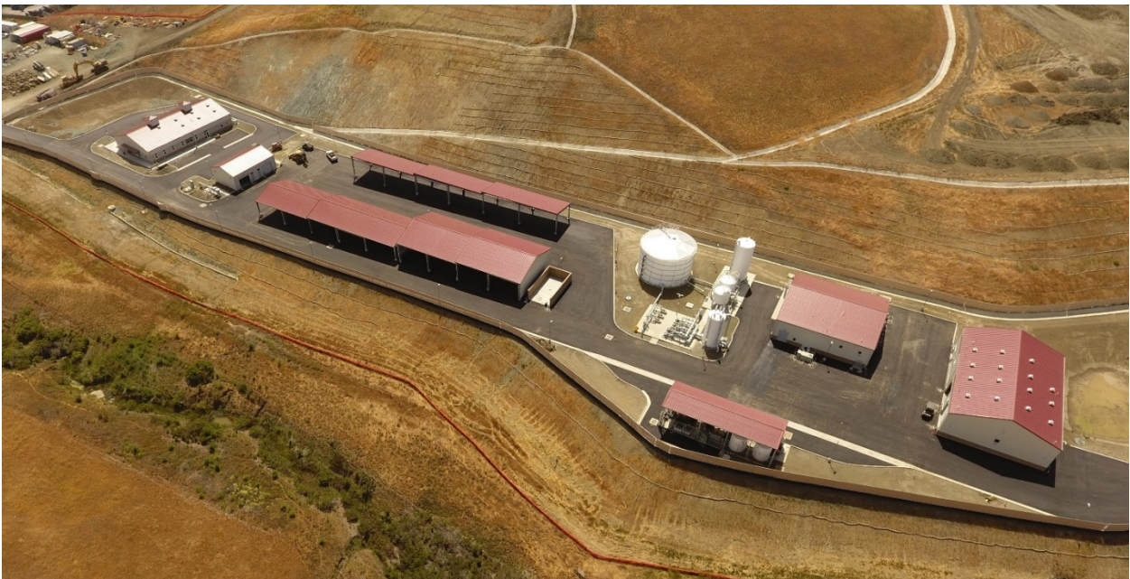
June 6, 2022 – Project Overview – Looking South
