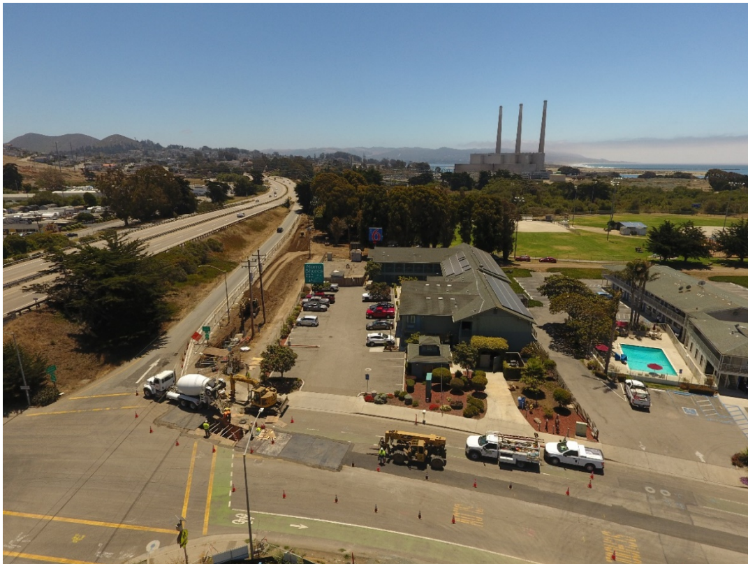
June 30, 2022 – Segments 1 & 2 (Joint Trench Installation within Caltrans ROW and Atascadero)
