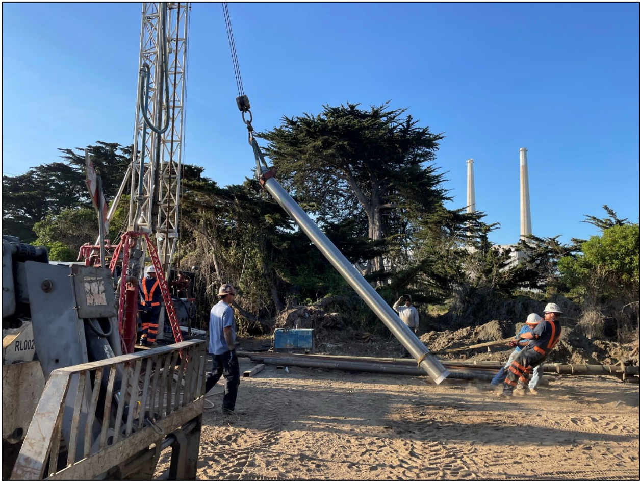
September 2, 2022 – Installation of the Pilot Injection Well Perforated Casing
