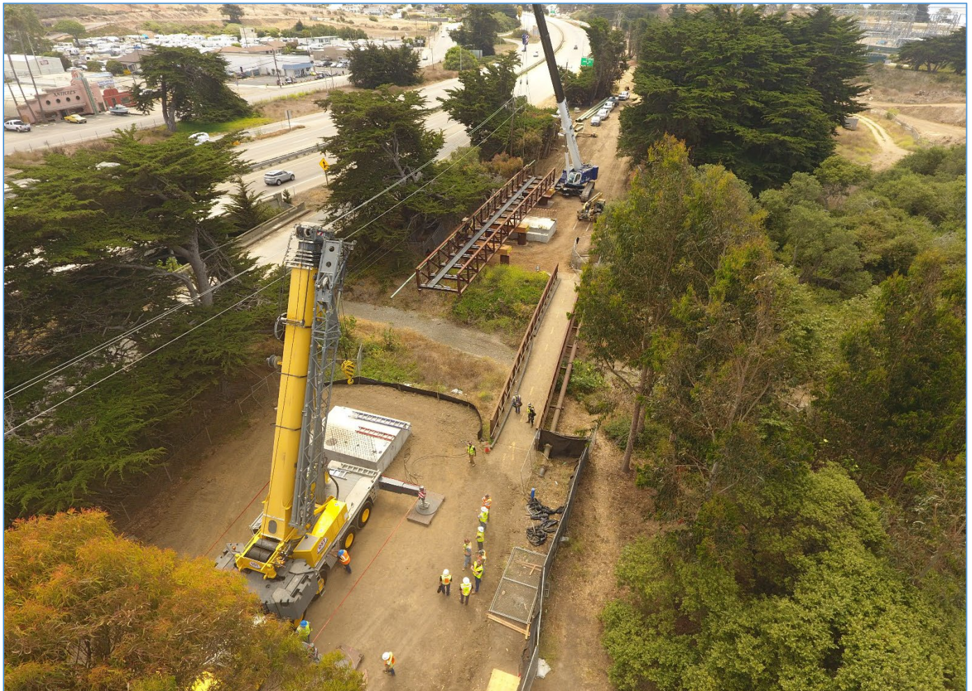
August 1, 2022 – Setting Utility Bridge over Morro Creek
