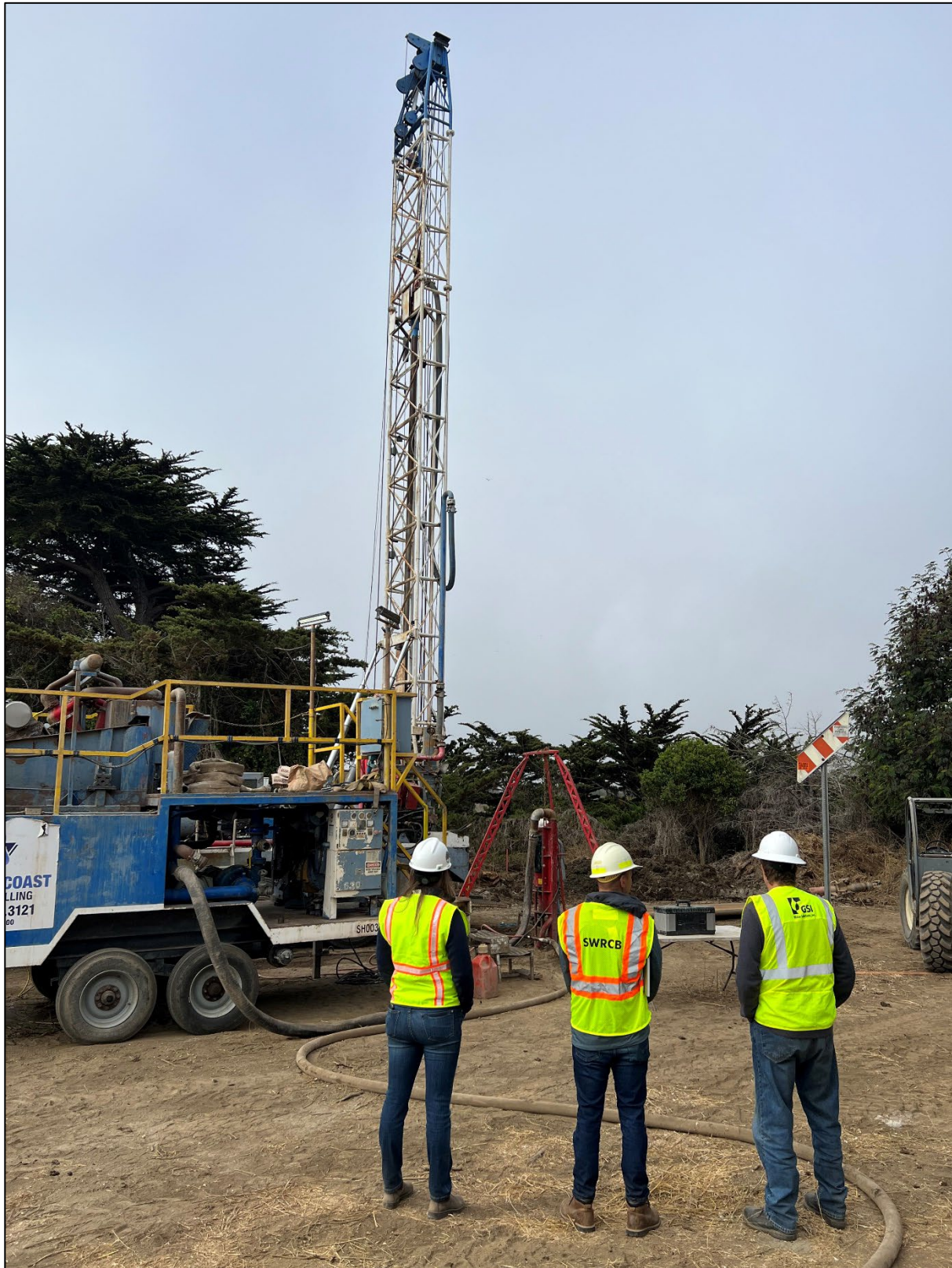
September 1, 2022 – Installation of the Pilot Injection Well Conductor Casing
