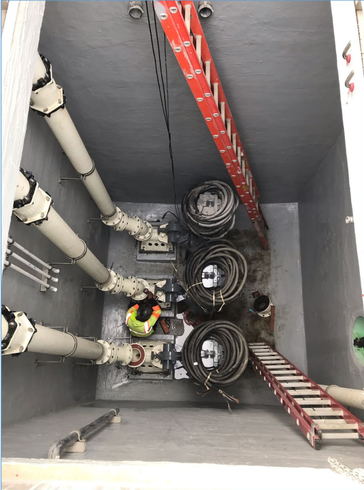
September 16, 2022 –Installing Piping and Pumps at Pump Station B wet well.
