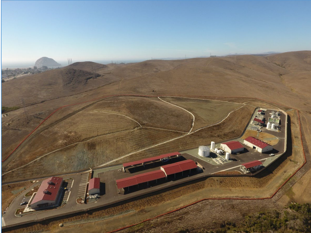
September 27, 2022 – Entire Site Overview
