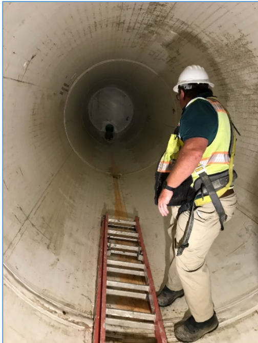
September 16, 2022 – Sealing Leaks and Holiday Testing Liner in Pump Station A Emergency Storage Tanks.
