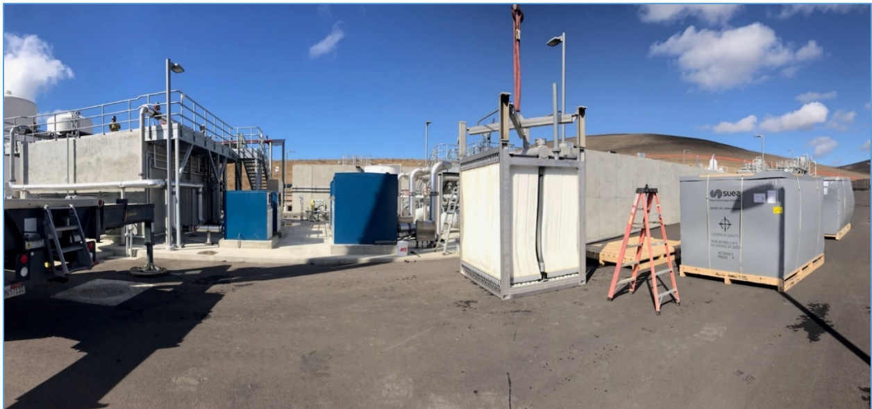
September 20, 2022 – Installing Suez MBR Cassettes
