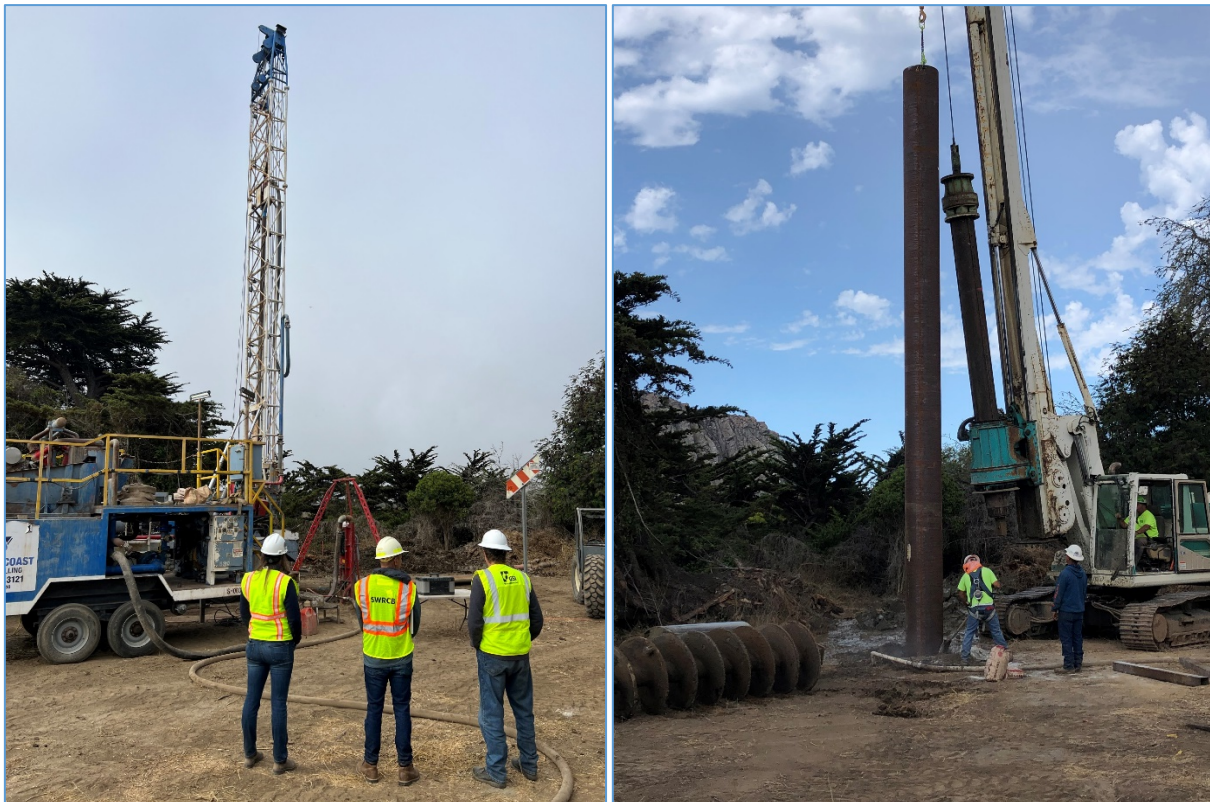
September 1, 2022 – Installation of the Pilot Injection Well Conductor Casing
