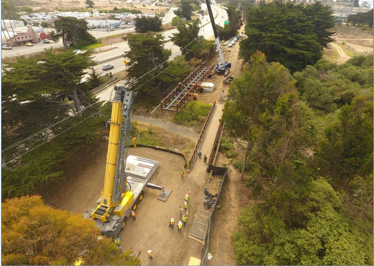
August 1, 2022 – Setting Utility Bridge Over Morro Creek
