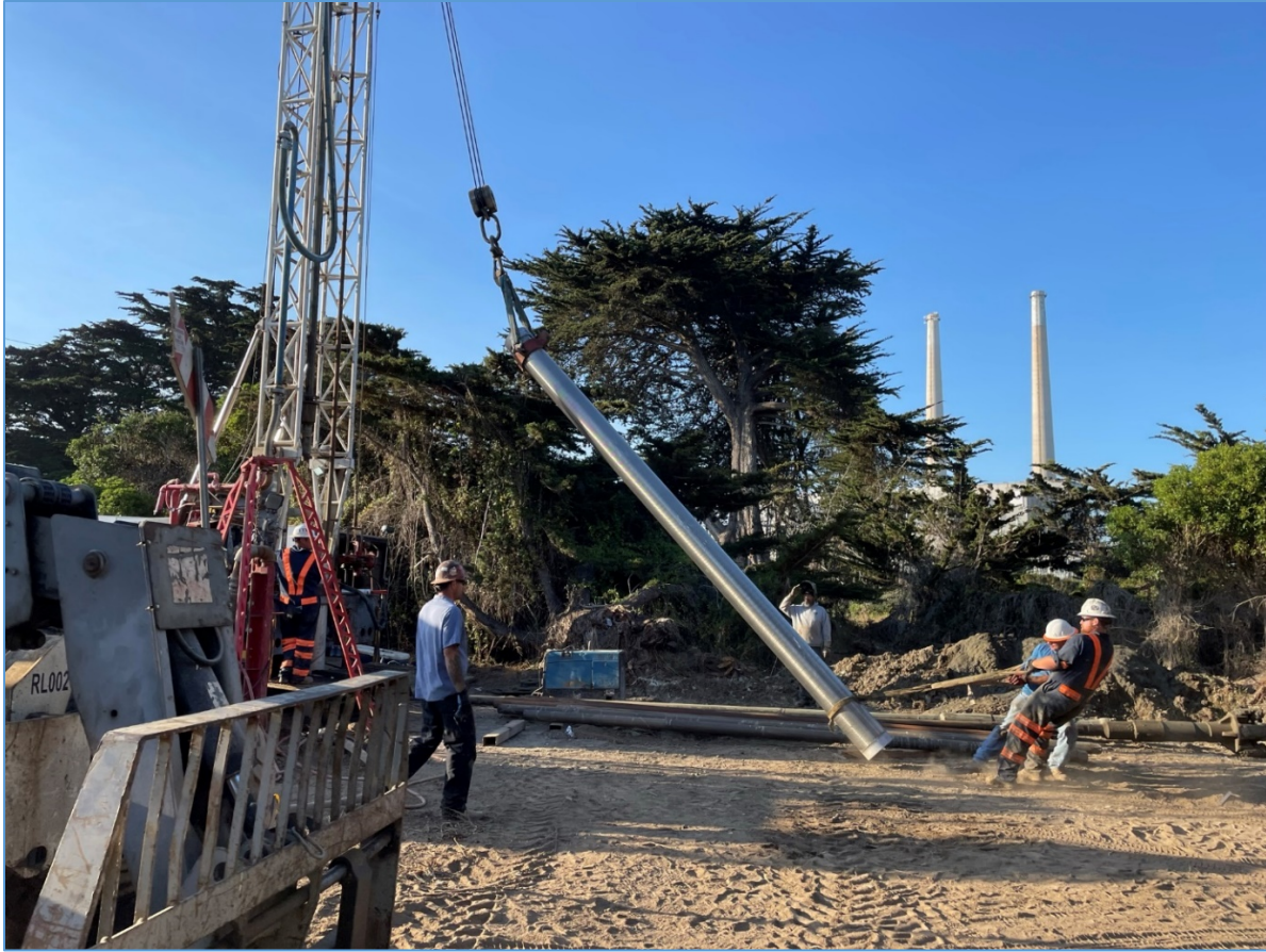
Installation of the Pilot Injection Well Perforated Casing
