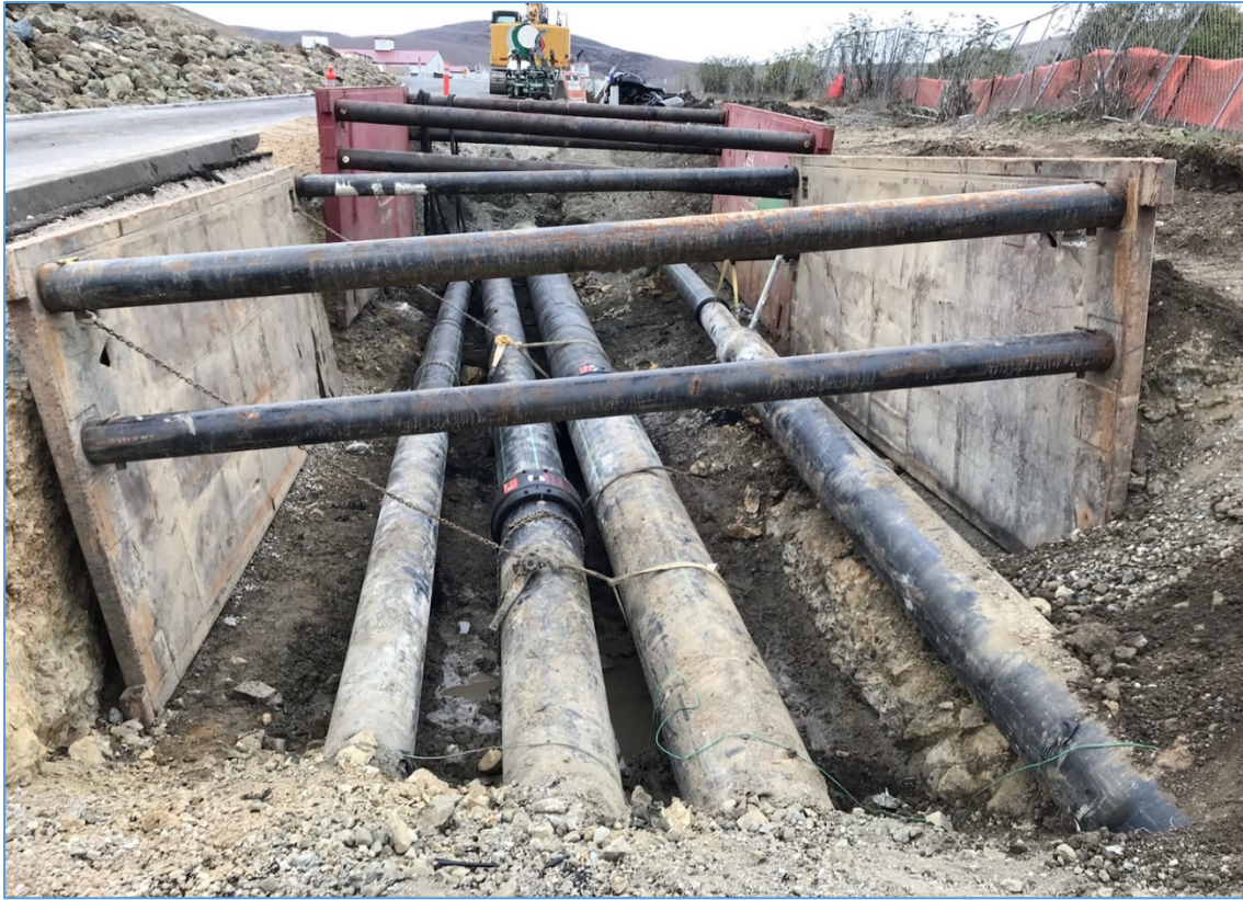
September 30, 2022 – Piping Connections Completed between Conveyance Project and WRF Site.
