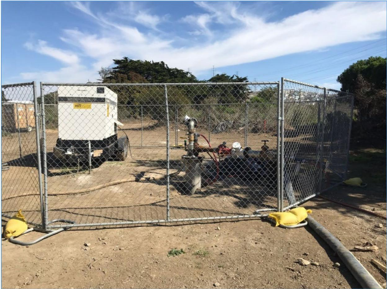
October 2022 – Pilot Injection Well completed with groundwater injection testing in progress.
