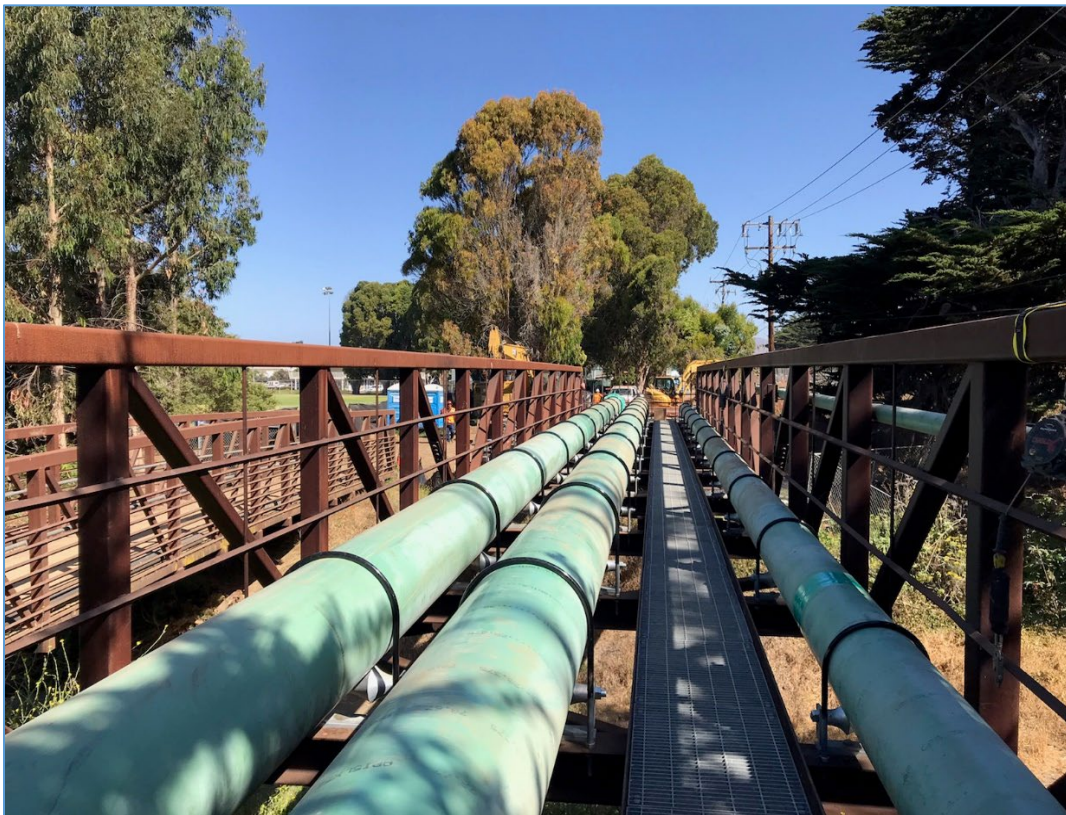
October 2022 – Utility Bridge Looking Over Morro Creek.
