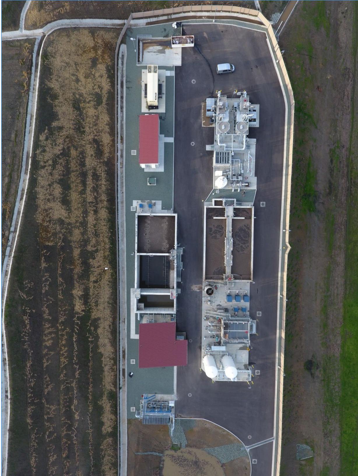
July 27, 2022 – Looking down at WRF Site (north site wastewater facilities).
