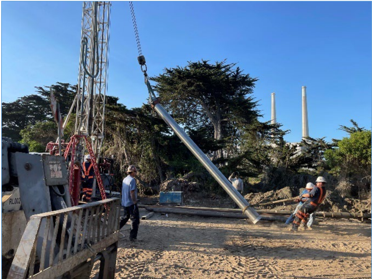
August 2022 – Pilot Injection Well Construction.
