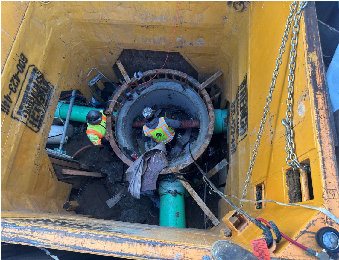
Nov 2022 – Constructing New Diversion Manhole Near Pump Station A.
