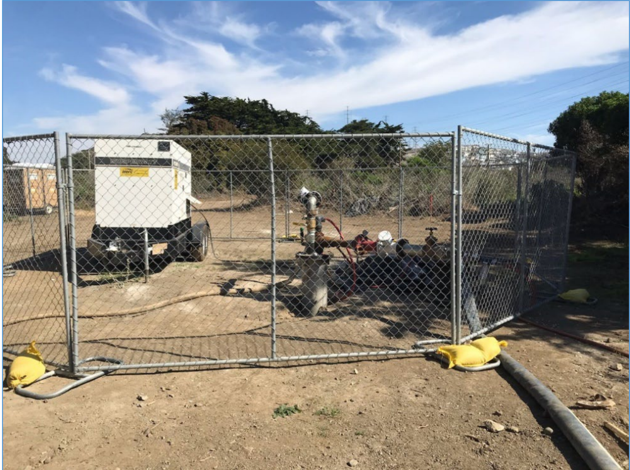
October 2022 – Pilot Injection Well Completed and Ready for Testing.
