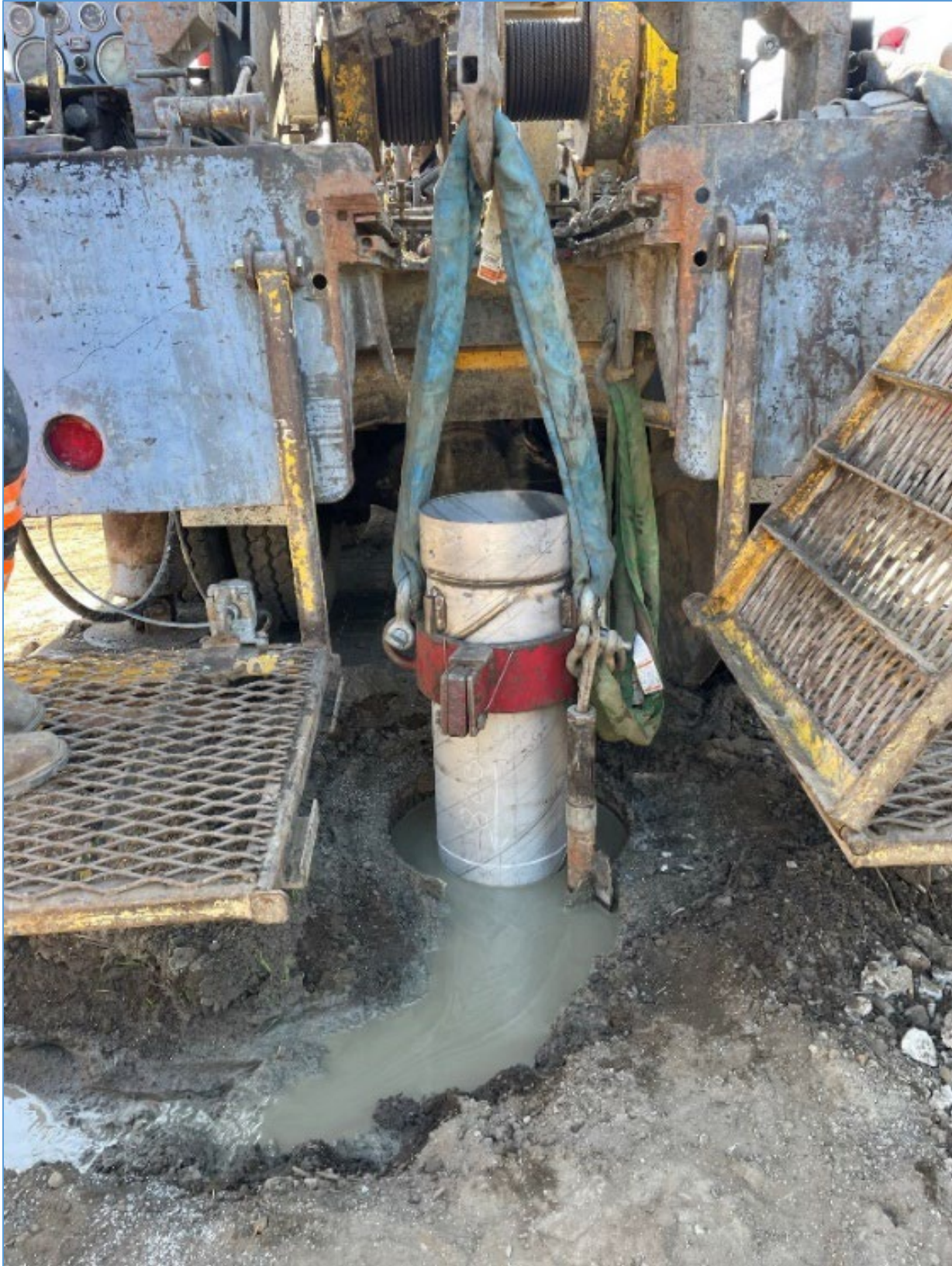
August 2022 – Pilot Injection Well Construction.
