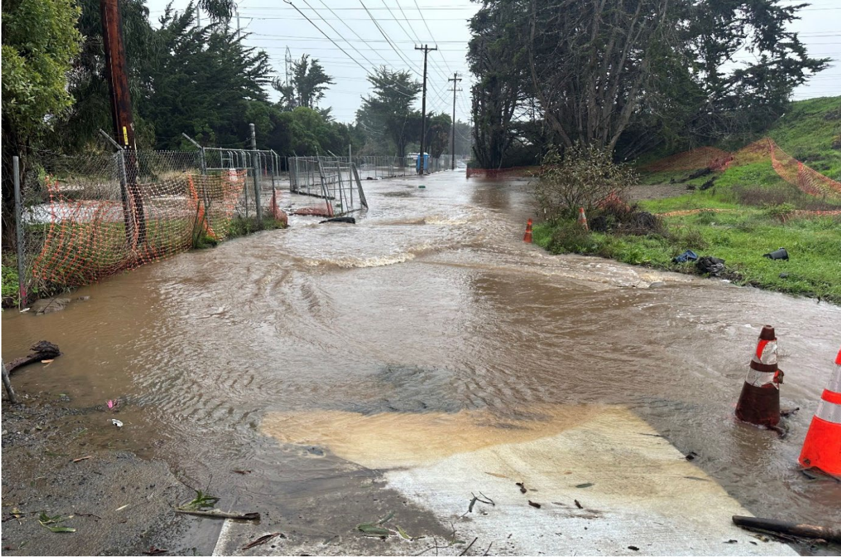
January 2023 – Flooding Along Bike Path
