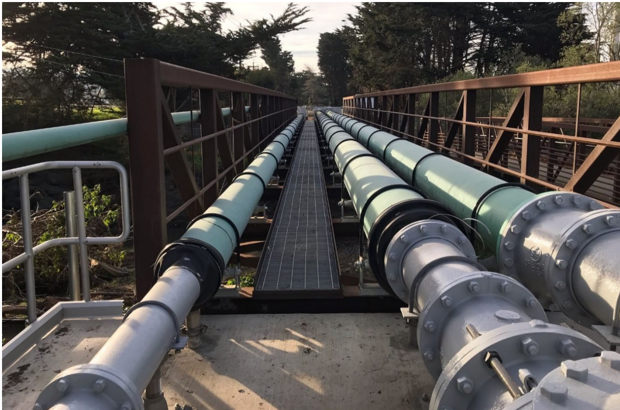
March 2023 – Completed Morro Creek Utility Bridge
