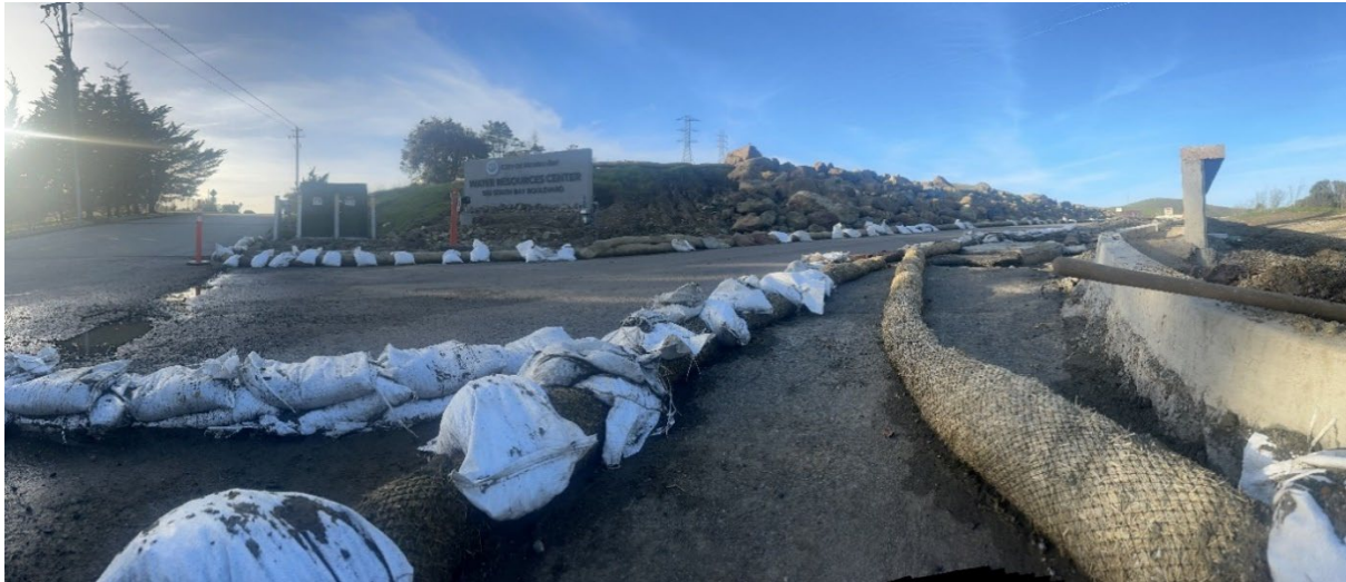
February 2023 – SWPPP BMPs at WRC Entrance in Preparation of Winter Storms
