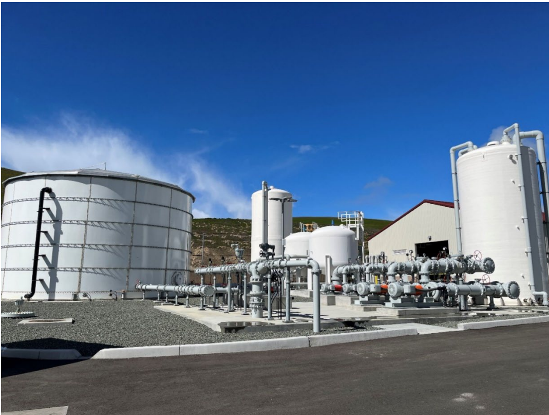
February 23, 2023 – Completed IPR Pump Station
