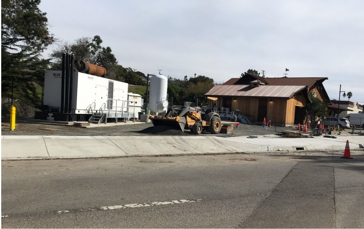
February 2023 – Pump Station B Fine Grading
