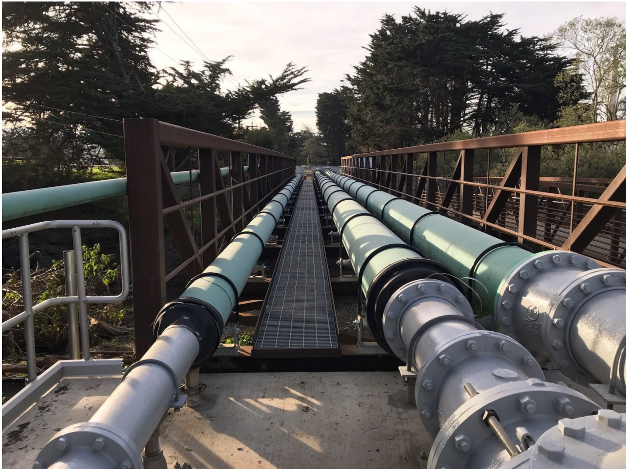
March 2023 – Completed Morro Creek Utility Bridge
