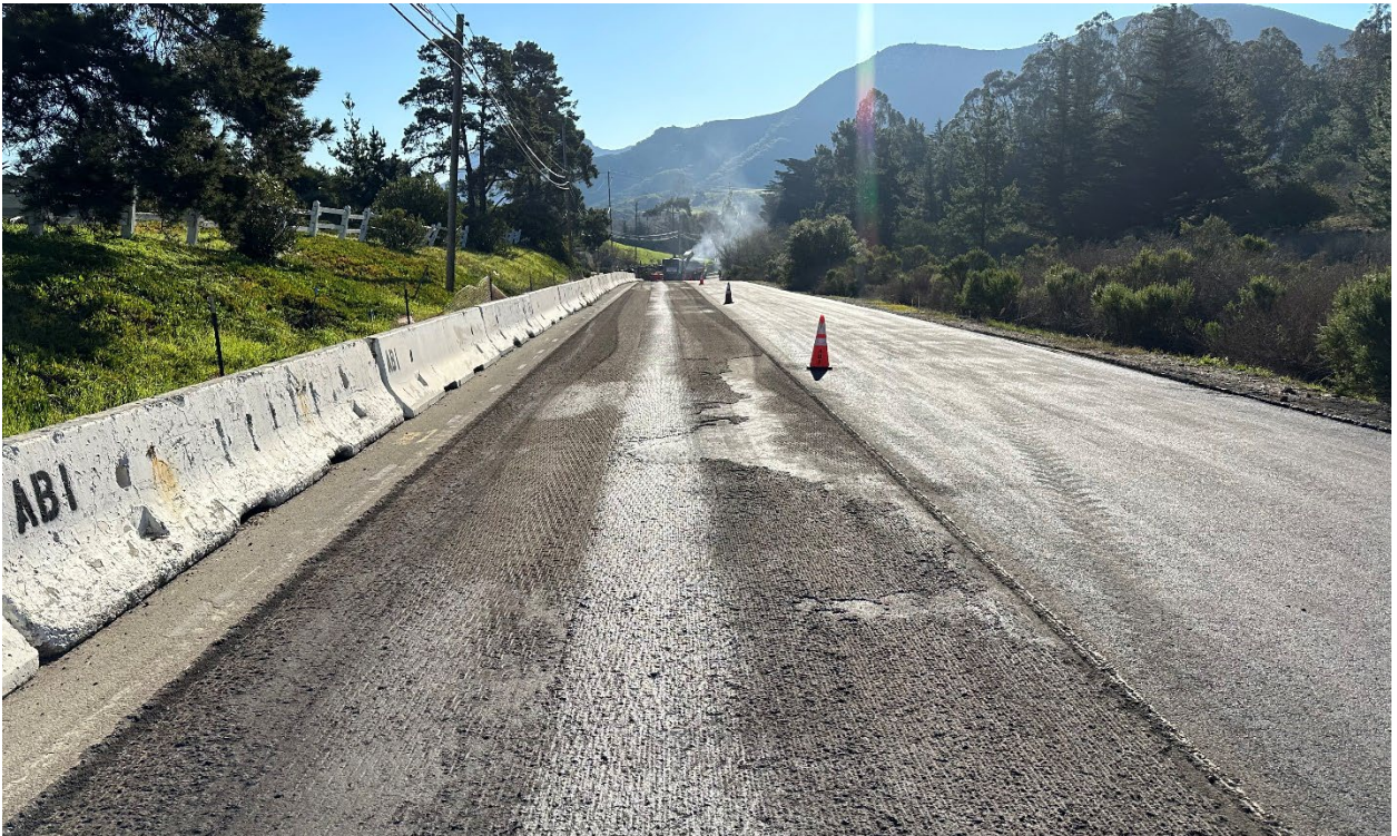
February 2023 – Quintana Road Paving
