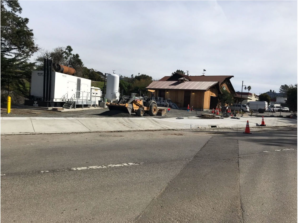
February 2023 – Pump Station B Fine Grading
