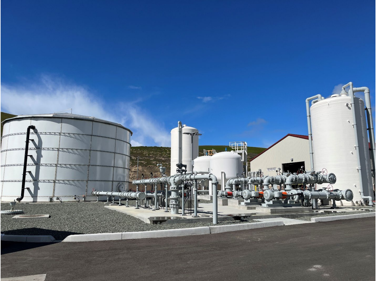
February 23, 2023 – Completed IPR Pump Station.
