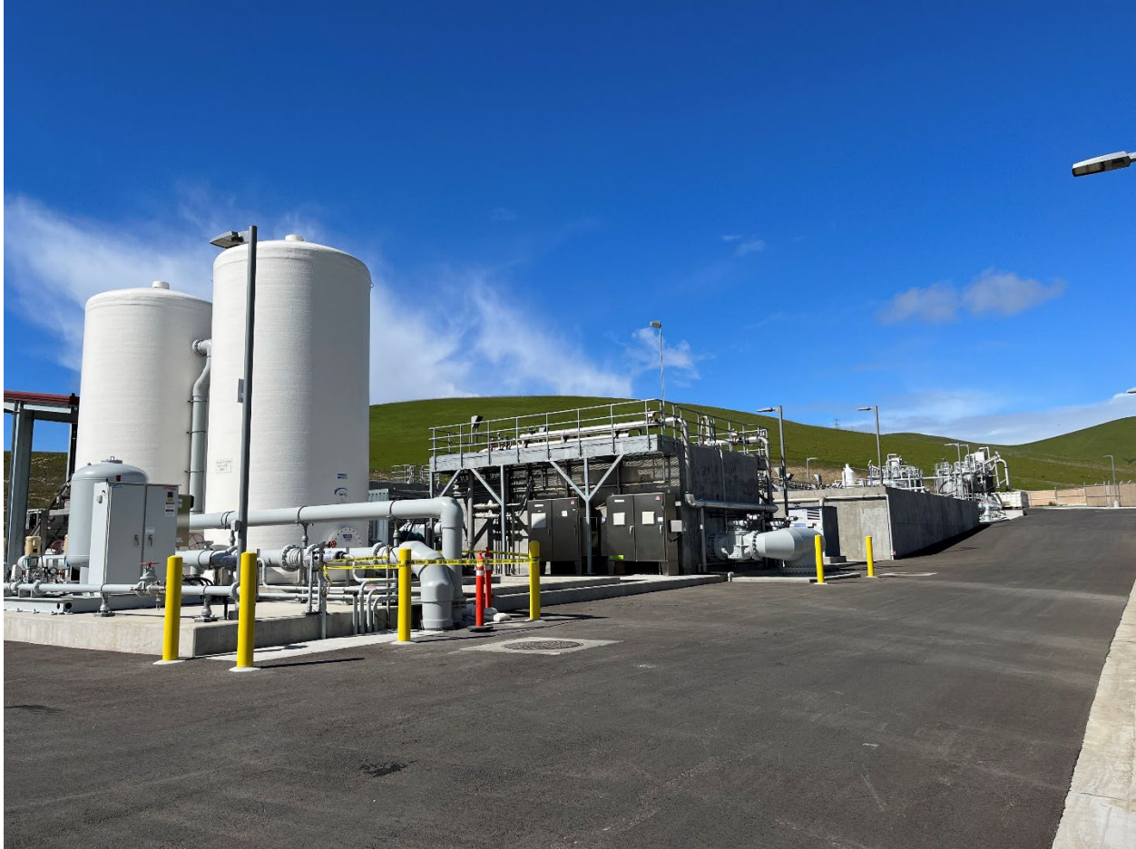
February 23, 2022 – Completed and Operational Headworks and Fine Screens.
