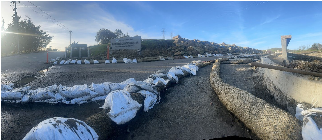
February 2023 – SWPPP BMP's at WRC entrance in preparation of February Storms
