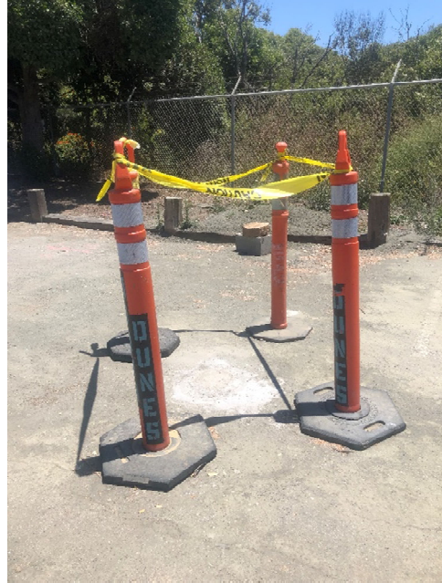
Well Site after Coring and Filling (SB #7)
