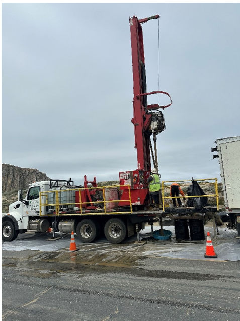
Well Site Coring – Sonic Boring No. 8 (SB No. 8)
