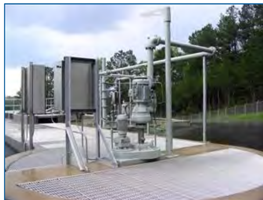
Figure 4-3 PistaGrit® Vortex Grit Removal System (Smith & Loveless)
