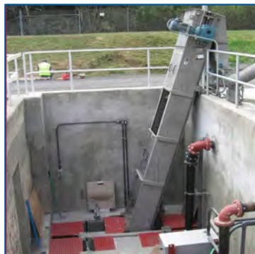
Figure 4-2 Mahr® Bar Multi-Rake Bar Screen
