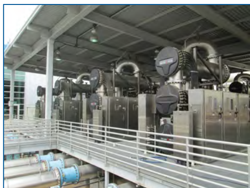
Figure 4-7 UV AOP at OCWD's GWRS Facility (UV Expansion Designed by B&V)
