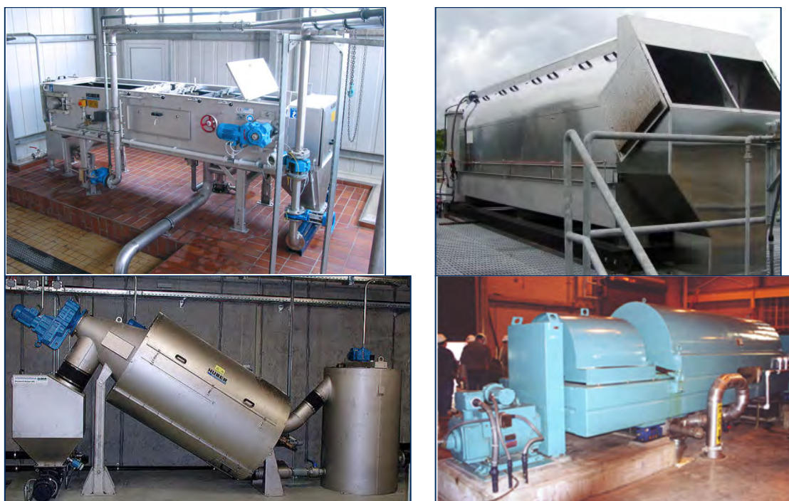
Figure 5-1 Four Suitable Sludge Thickening Technologies: Gravity Belt Thickener (Huber Corporation, 2013), Rotary Drum Thickener (Parkson, 2013), Screw Thickener (Huber Corporation, 2013), and Thickening Centrifuge
