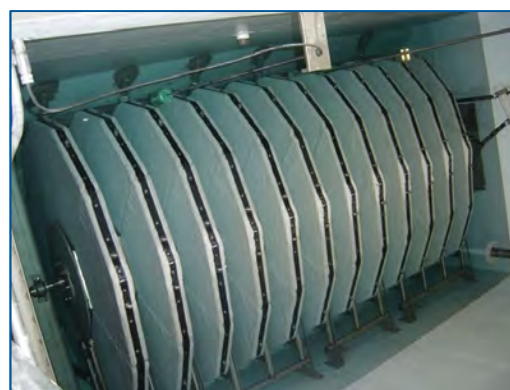
Figure 4-6 AquaDisk® Disc Filter (Aqua-Aerobic Systems)
