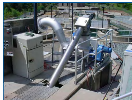
Figure 4-1 CleanFlo® Spiral Screen & Wash Press (WestTech)
