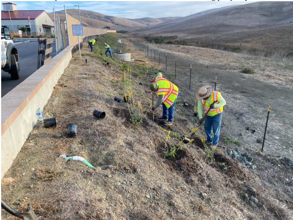
Photo 4. View of site entrance looking north while crews installed replacement plants in October 2023. Several substitutions occurred including the use of California goldenrod shown here.
