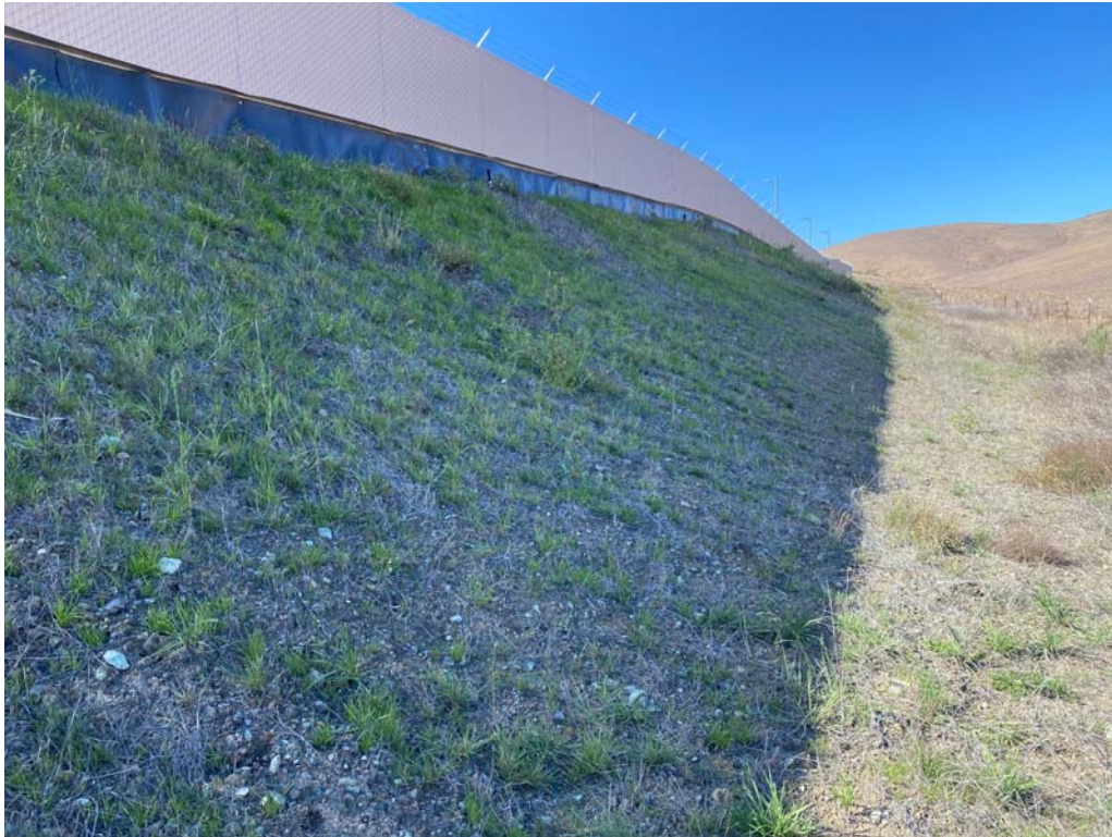
Photo 7. View of Photo Point 3 area looking northerly in between container planting areas showing establishing native grasses applied via hydroseed. Supplemental irrigation has aided in plant growth throughout the REP area.
