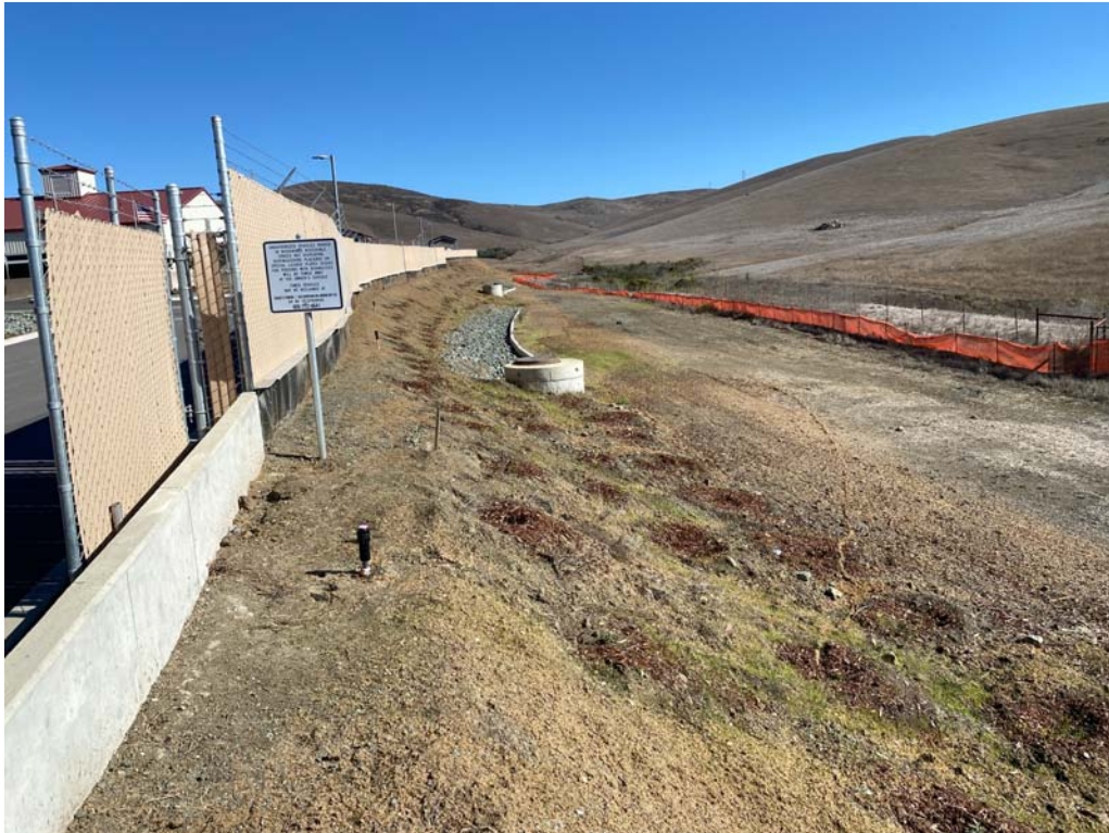
Photo 1. Northerly view of initial REP planting in September 2022. Due to a heat wave that occurred immediately after planting, over half of the container plants died. As a result, additional plant material was acquired and replanting occurred in October 2023.
