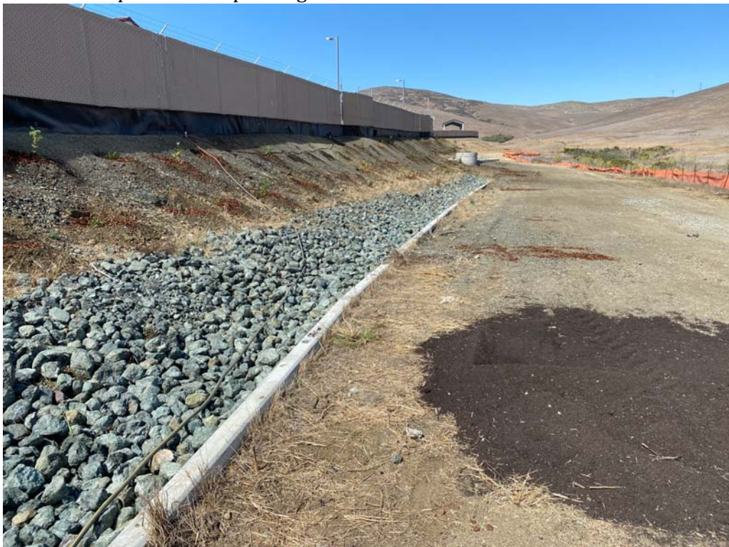
Photo 2. Compost and bark mulch were used in each planting area to help with plant establishment. View of the southern container plant area adjacent to a drainage dissipator.
