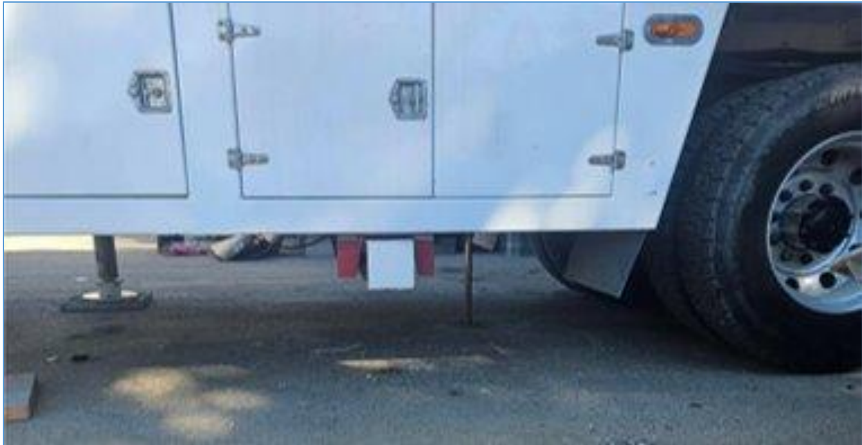
Figure 4 Hydrogeological Investigations (CPT Corings) for Injection Well Siting
