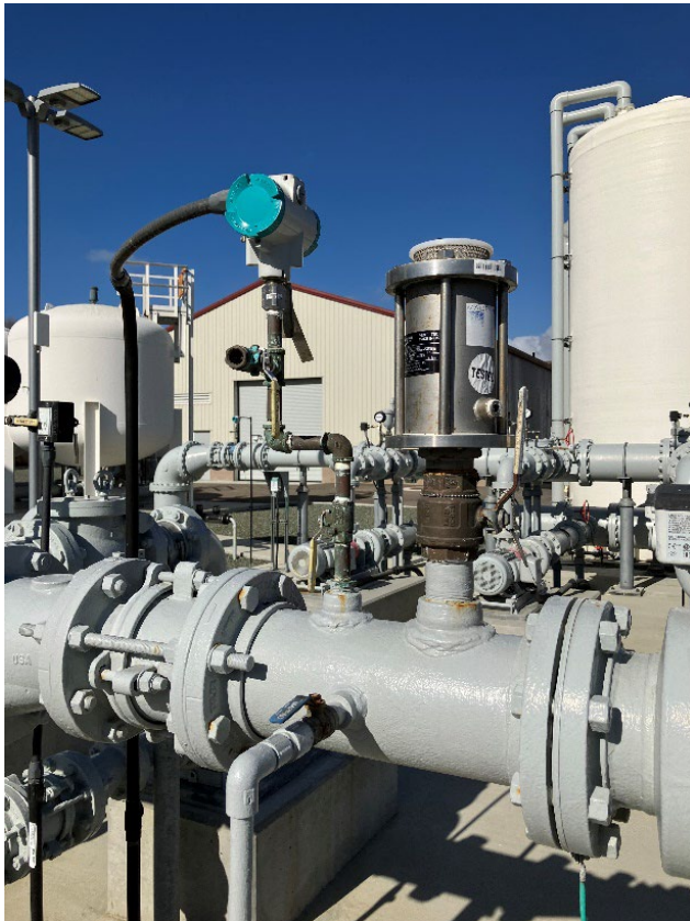
Figure 2-3 Vent-Tech SDG Valve on IPR Pump Station Discharge Header
