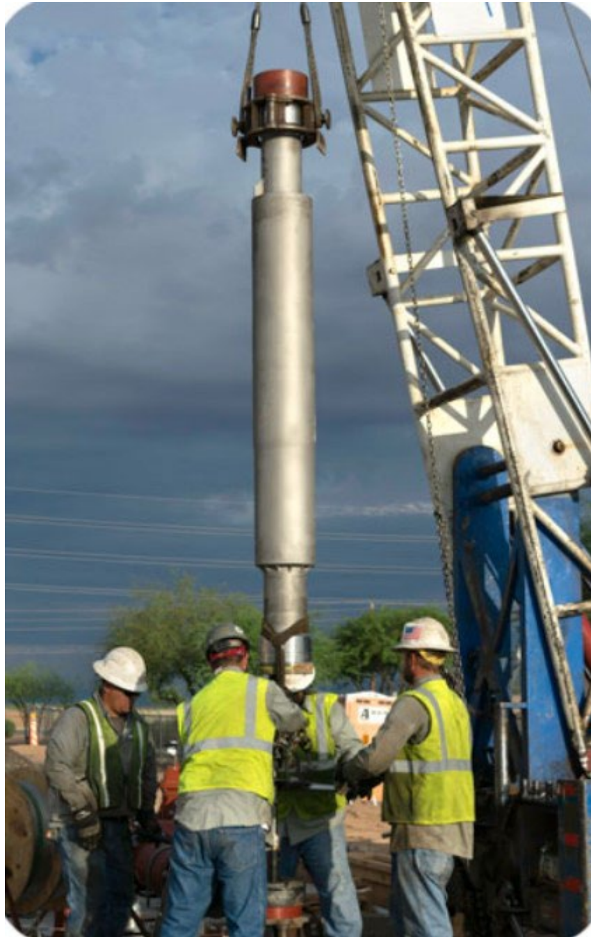
Figure 6-3 Baski InFlex Valve Installation
