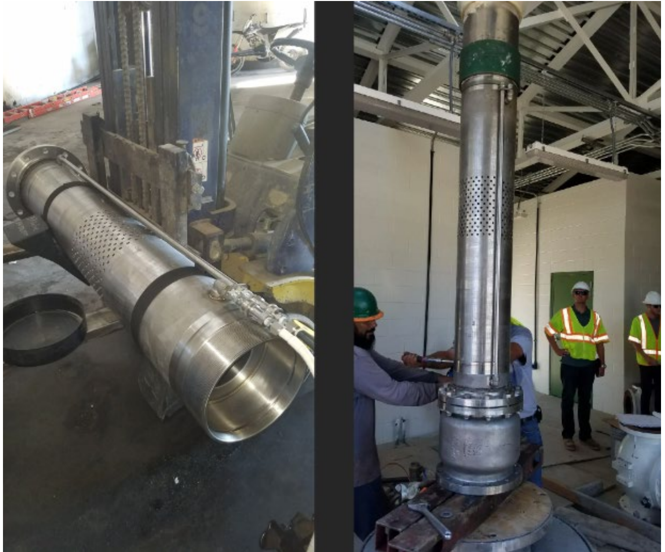
Figure 6-4 3R Valve and Installation
