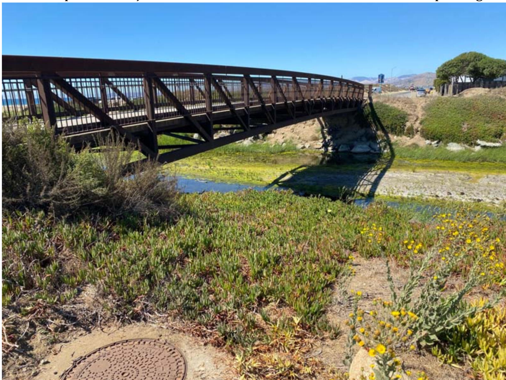
Photo 14. Northerly view of the existing bridge over Morro Creek that is in Segment 7A. In this location, the RWF pipeline would be installed in an existing pipeline under the creek or attached to the bridge to avoid impacts to riverine, riparian and wetland habitats.
