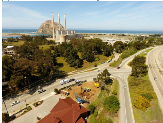
Lift station construction on Main Street - April 2021
