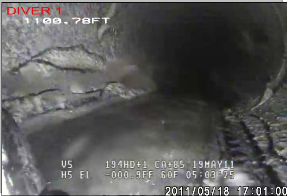
Figure 9 - Joint Seal Partially Detached from Pipe and Downstream Portion of the Bend
