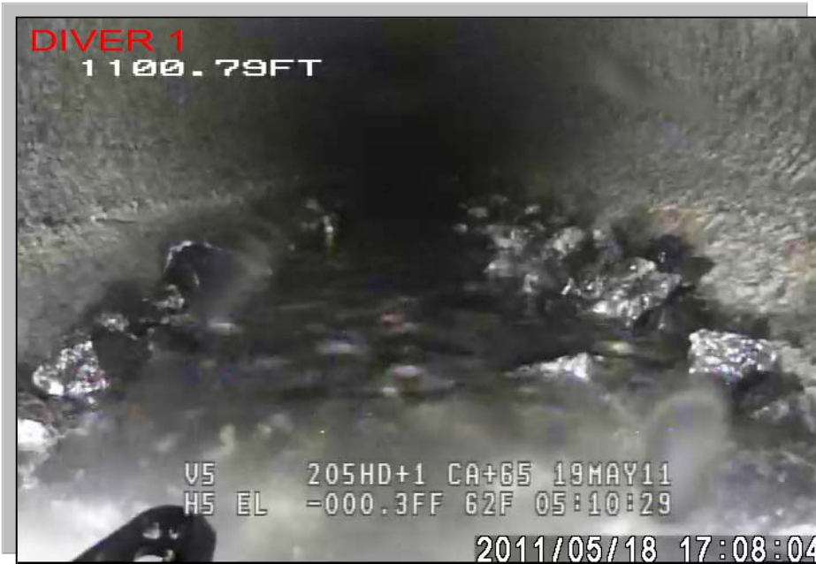
Figure 12 - Typical Debris on Invert
