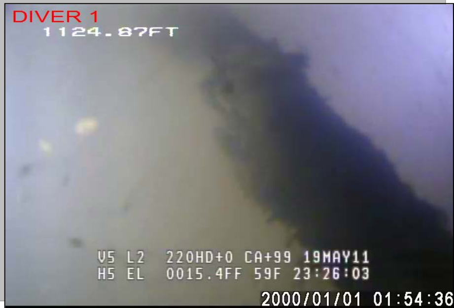
Figure 14 – Seal Debris Partially Blocking Pipe
