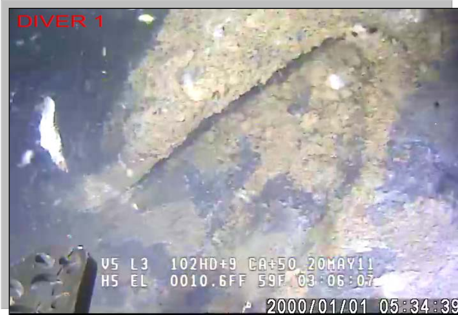
Figure 16 - Seal Loose from Crown between 1300' and 1200'
