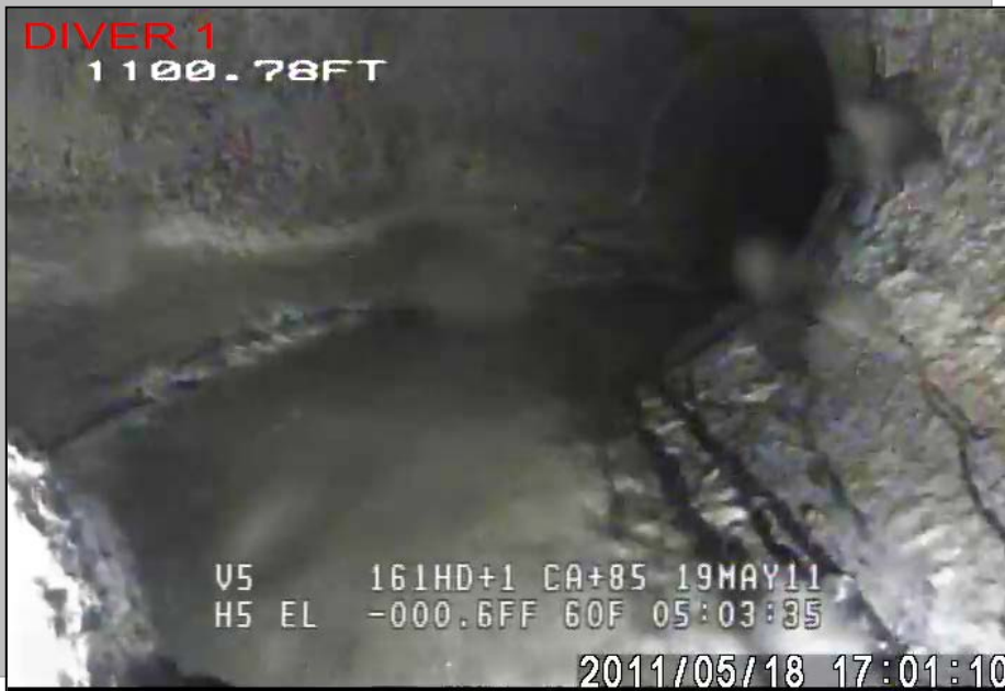
Figure 10 - Bend in Pipe
