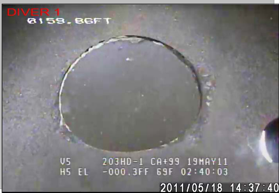
Figure 5 - Circular Plug in Crown of Pipe
