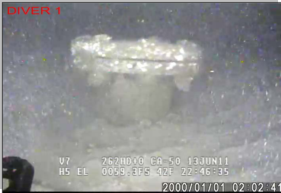
Figure 22 - Stand Pipe at End of Outfall
