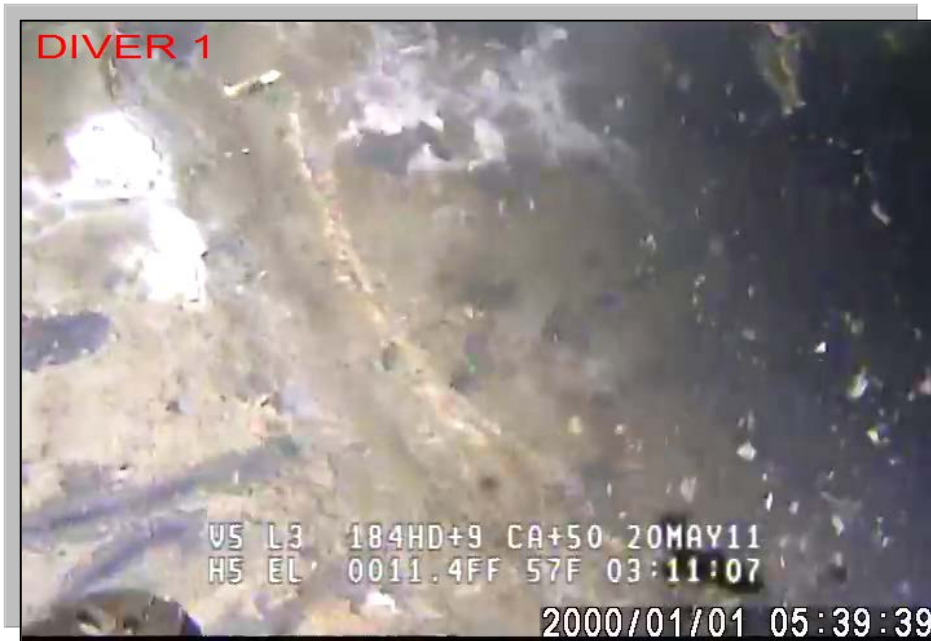
Figure 18 - Seal Missing from Joint between 1100' and 1068'
