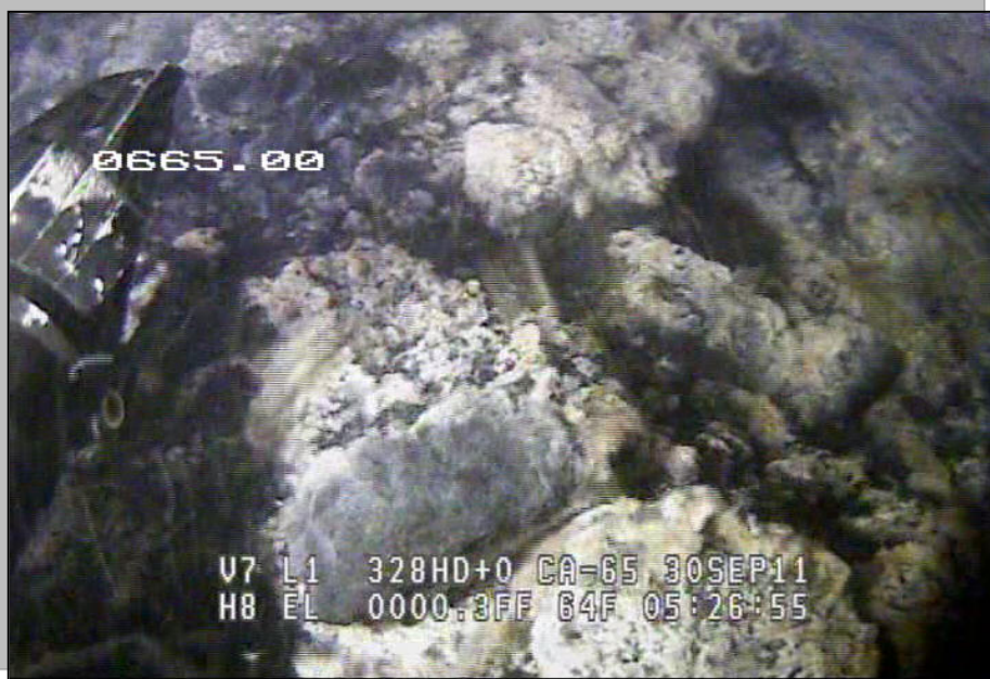
Figure 21 - Invert Debris at 665'
