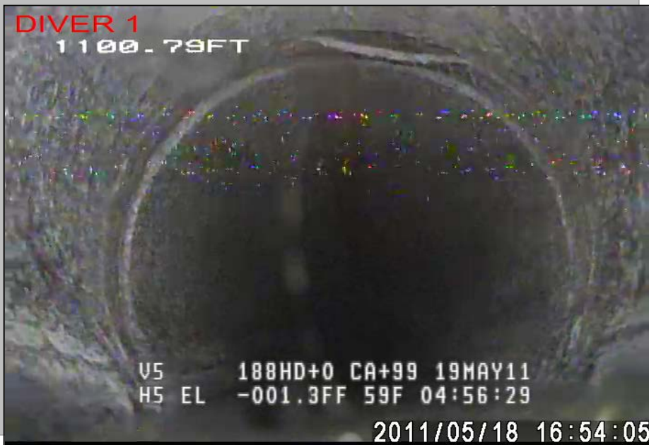
Figure 8 - Joint Seal Hanging from Crown
