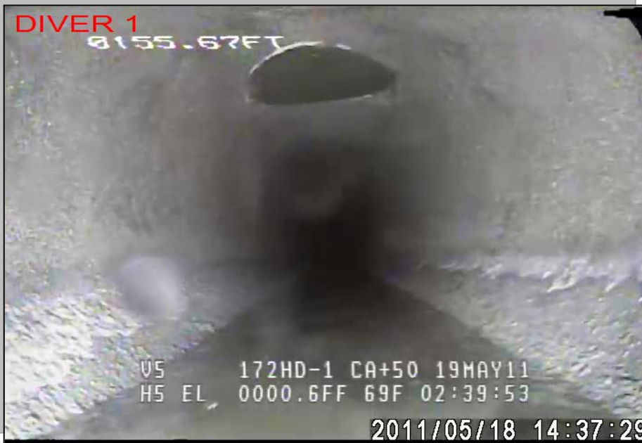
Figure 6 - Different View of Circular Plug in Crown at 155'
