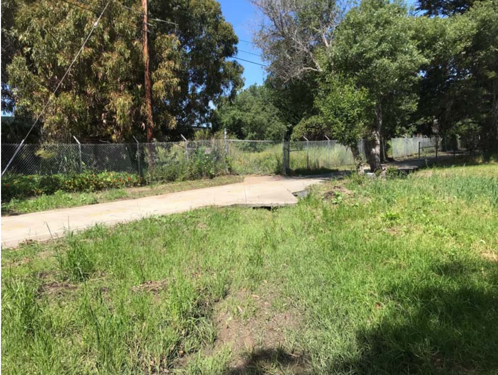
Photo 5. Easterly view of Drainage 1 at the bikepath concrete culvert that will be buffered 50 feet and jack and bore techniques used for pipeline installation to avoid impacts to the drainage feature.
