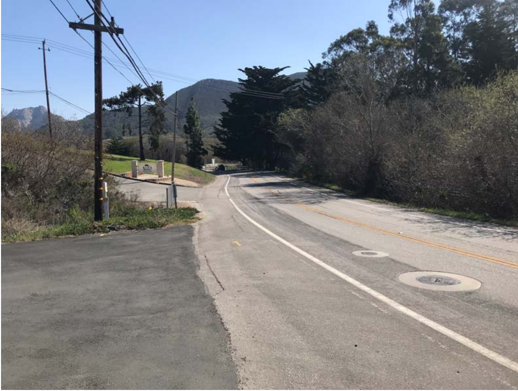
Photo 7. Easterly view of Drainage 2B work area along Quintana Road. Willow riparian scrub present in the drainage feature will not be affected since work will occur in the disturbed road right of way.
