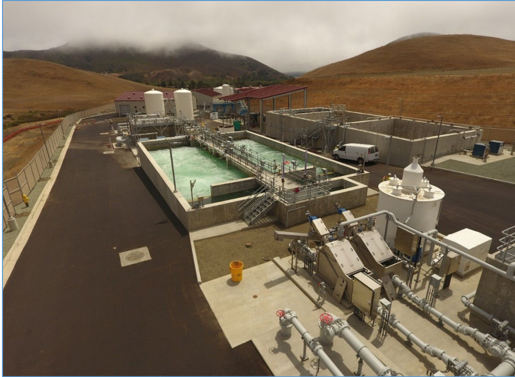
September 27, 2022 – Looking south (Fine Screens and Odor Control, BNR basin clean water testing)
