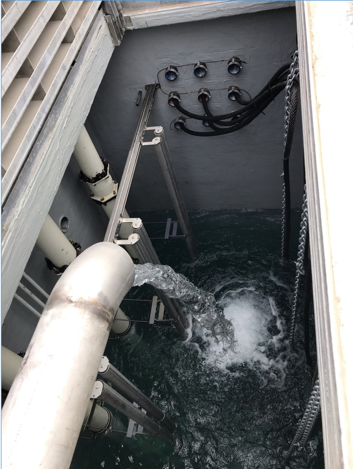
October 2022 – Clean water testing and flushing at Pump Station B wet well.
