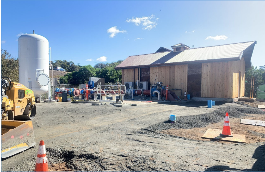
Nov 2022 – Pump Station B Electrical Building, Surge Tank, Discharge Piping, and site grading.
