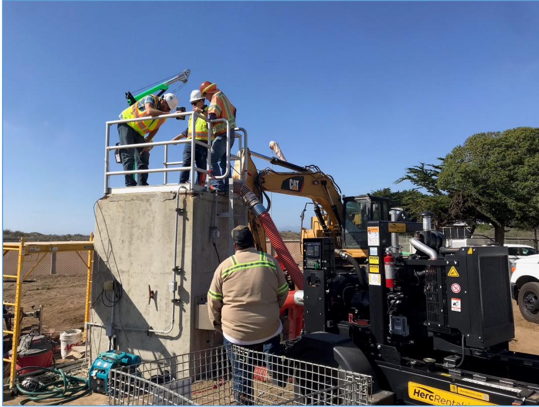
October 2022 – Clean water flushing new Brine Line at the City's Existing Ocean Outfall Box.
